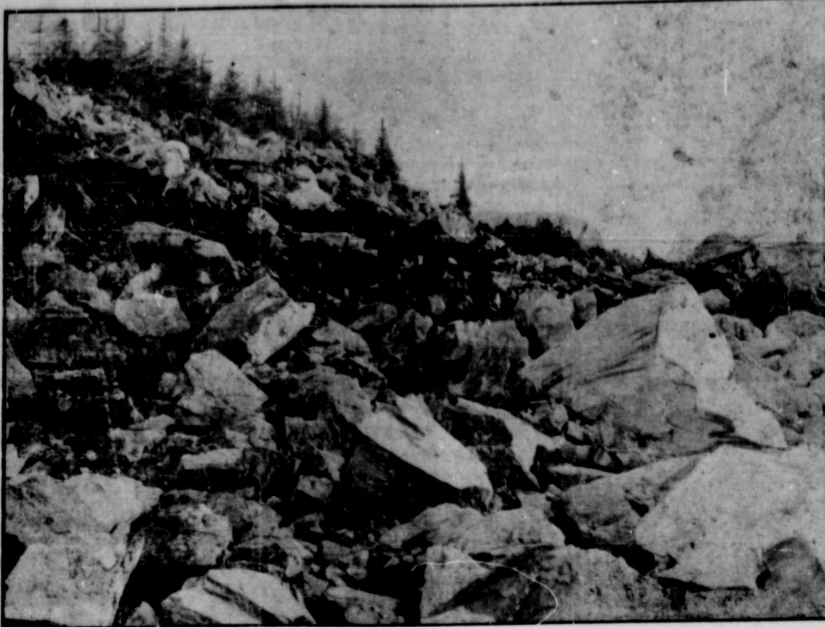
Above is a photograph reproduced showing the effects of one of the big coyotes fired on railway contract work in the city limits and similar to that fired the other week at Cameron Bay. Preparations are in progress for another big coyote at Hays Creek soon, also in connection with the dry dock shoreward operations.
