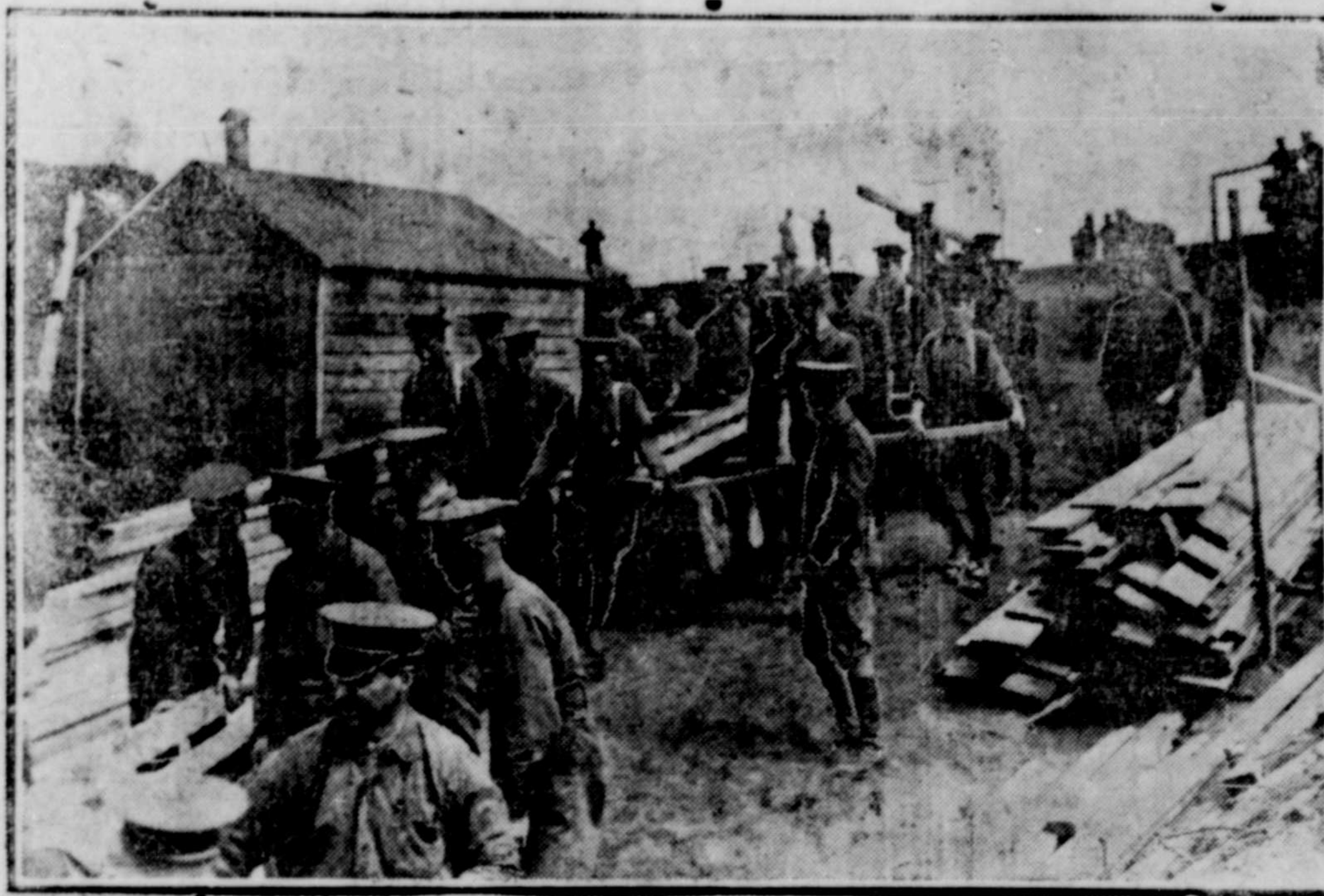
300 ROYAL CANADIAN ENGINEERS BUILDING A PONTOON.
