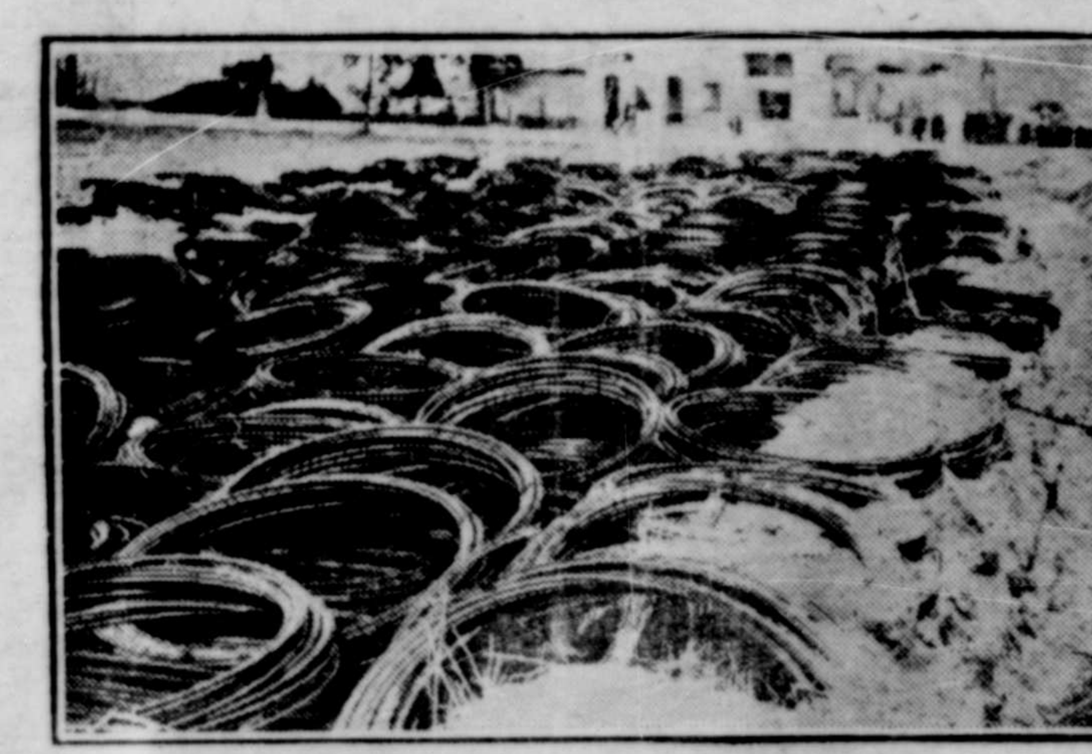
PROTECTION FOR GERMAN TRENCHES The Germans have found a new plan for the protection of their soldiers in the trenches. Coils of wire are placed before the trenches and when a shell falls they prevent the fragments from spreading to the trenches.
