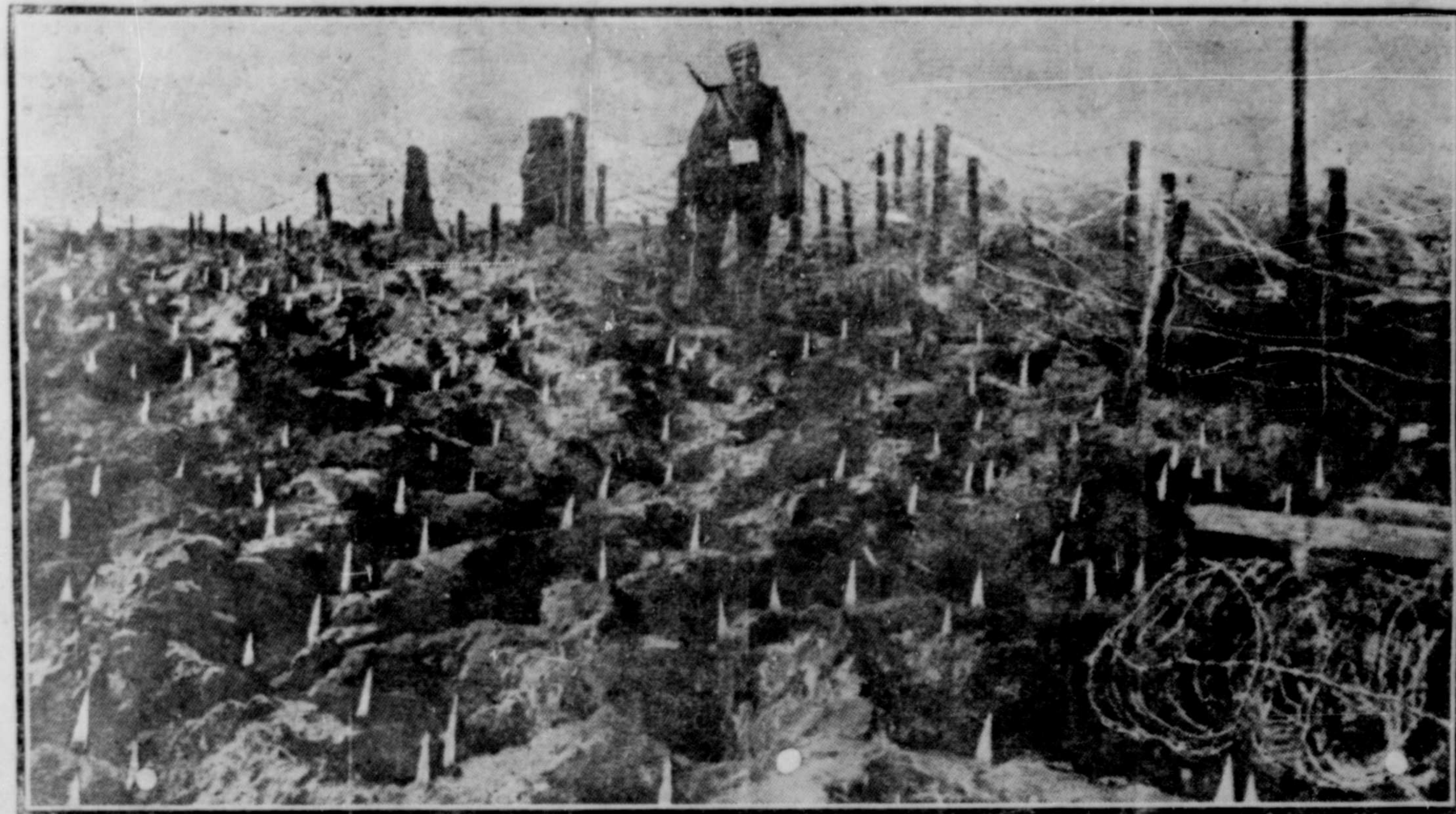
AUSTRIAN ENTANGLEMENTS TO IMPEDE ENEMY —The picture shows the pitfalls, surrounded by sharp spikes which the Austrians construct near their fortresses. The barbed wire on the right of the picture is heavily charged with electricity which would prevent any number of soldiers from gaining access to the fortress.
