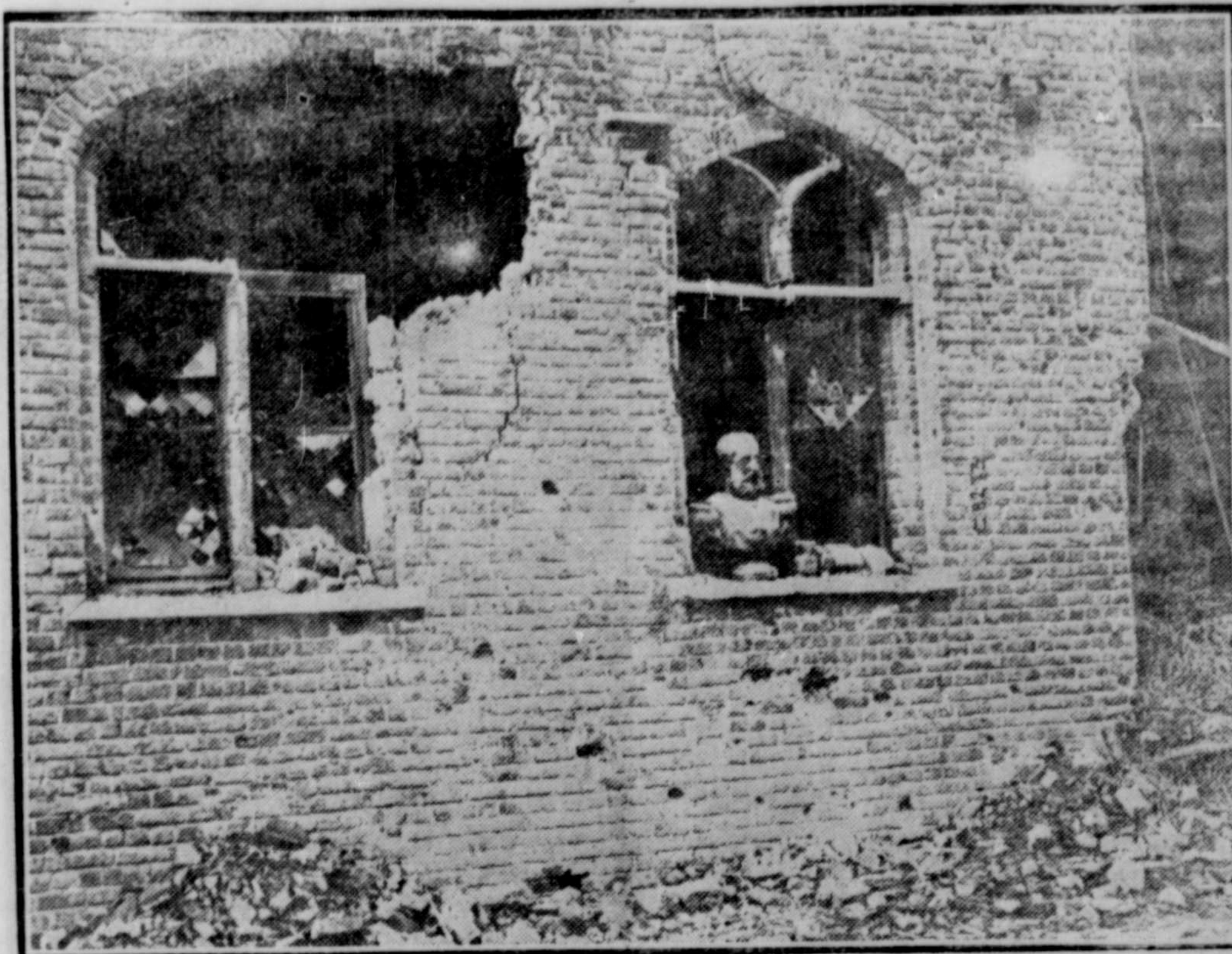
A WALL OF YPRES MUSEUM.—The Museum of Ypres has been entirely destroyed. One of the walls of the famous structure shows what the bombardment did.
