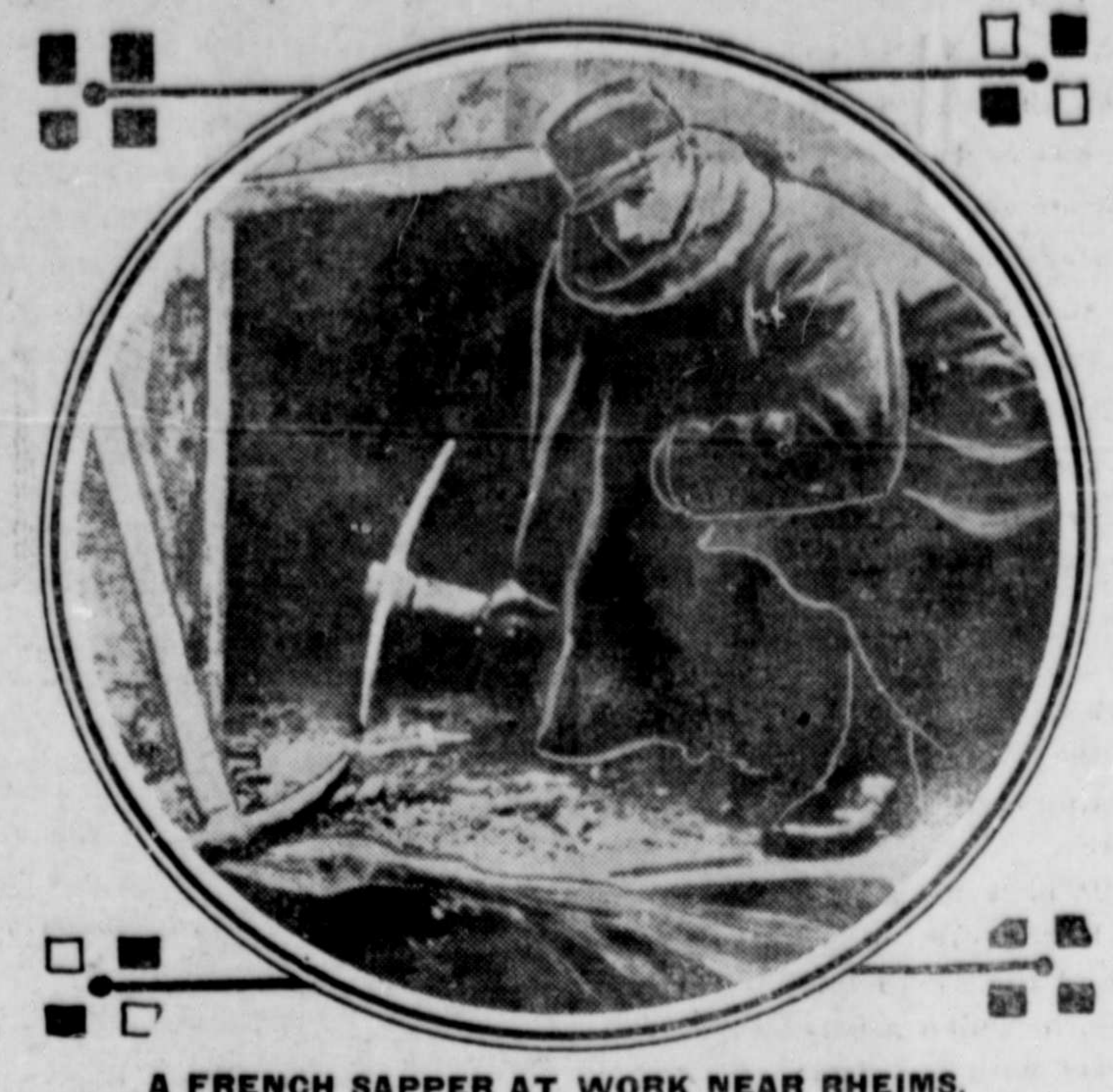
A FRENCH SAPPER AT WORK NEAR RHEIMS. This form of warfare, burrowing beneath the trenches of the enemy and blowing them up, has been used with telling effect by the French around Rheims.
