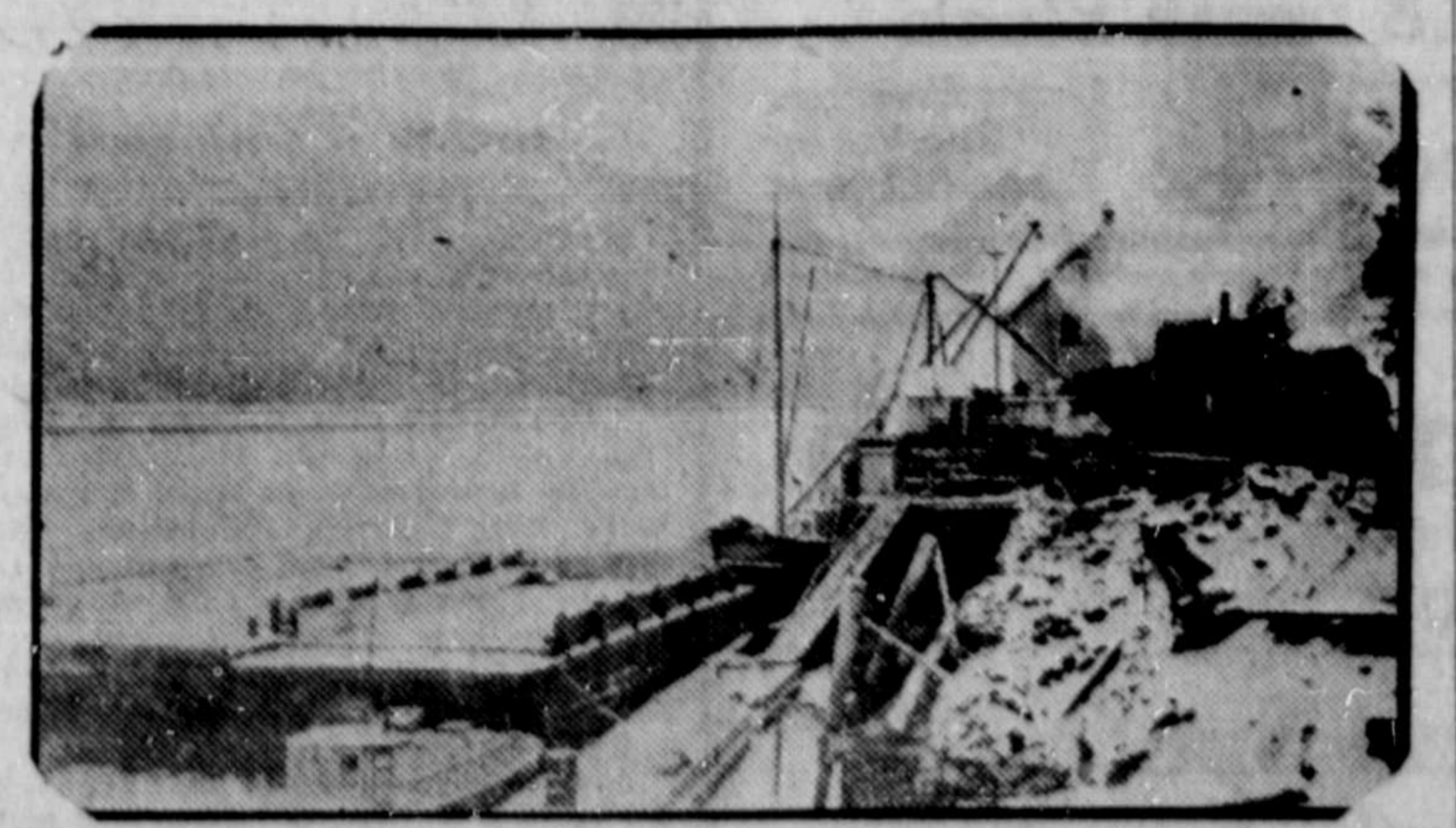
DOLLY VARDEN WHARF from which the Taylor Mining Co. ships the rich ore that comes 18 miles by rail to Alice Arm from mine.
