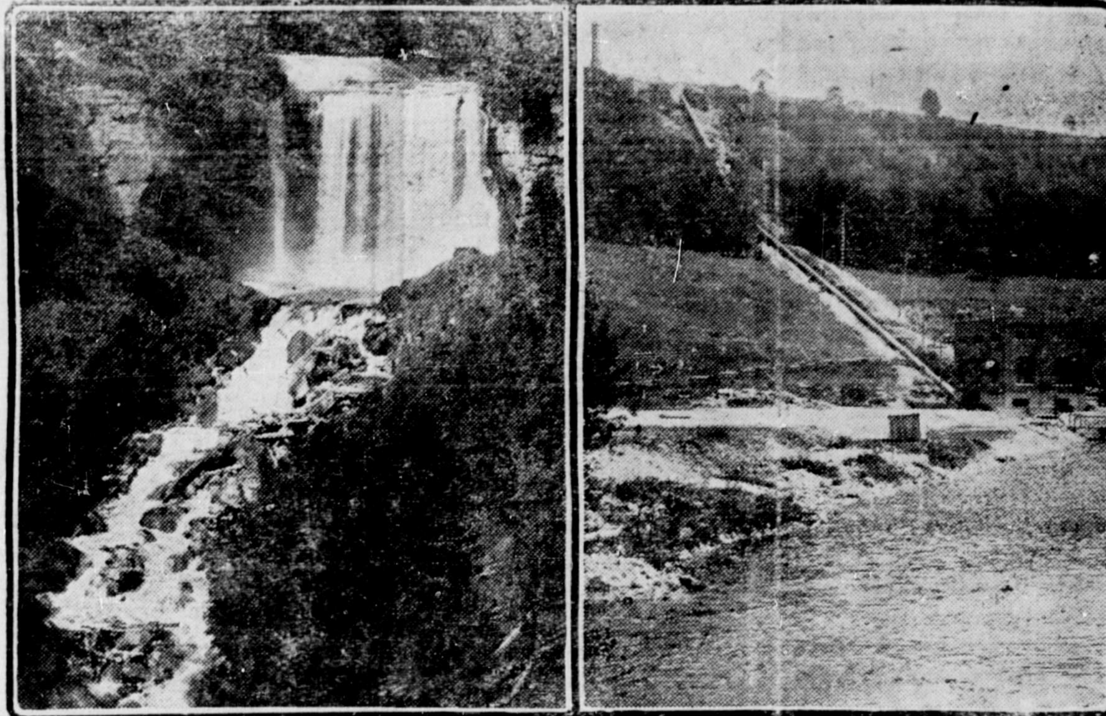
WONDERFUL CANADIAN ENGINEERING FEAT.—The two views show Tugenia Falls, near Flesherton, Ont., before and after the Beaver river was "squeezed" into a single pipe by the hydro electric engineers for developing power. The pipe delivers the accumulated flow from 2,500 acres at the power house, a drop of 520 feet, the second largest in Canada, exceeding that of Niagara.
