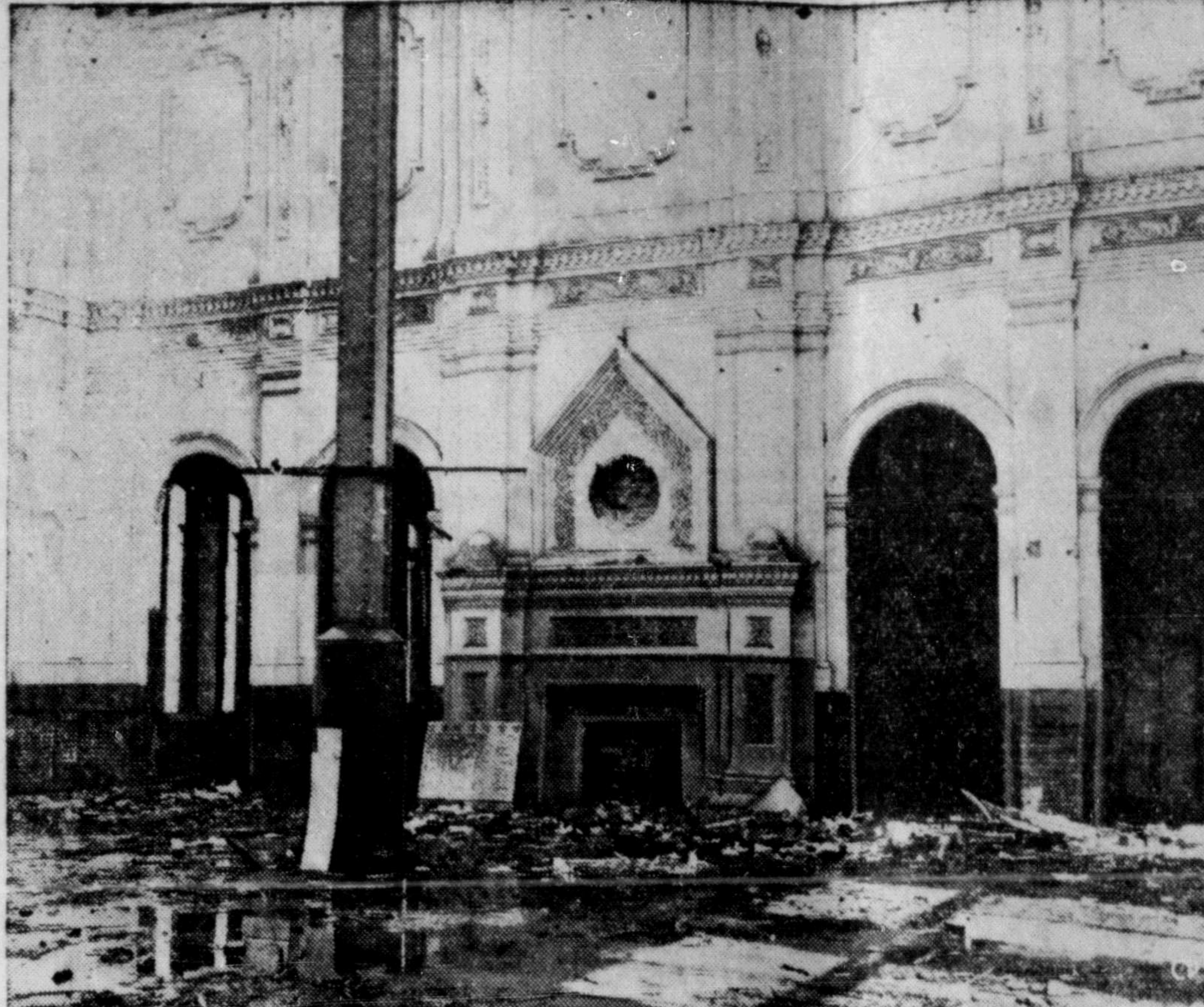
LANDMARK DEMOLISHED—Two major fires, causing millions of dollars damage, failed to wipe out historic Bonaventure station in Montreal, but demolition men now are slowly tearing it down. The Canadian National Railways terminal, once a railway showplace, handed millions of travellers since it was built in 1887. Shown is the interior of the concourse. A tottering steel pillar holds up the roof as ornate plaster frescoes, the huge fireplace and old plaques and carvings await the pick and sledge. (CP PHOTO)
