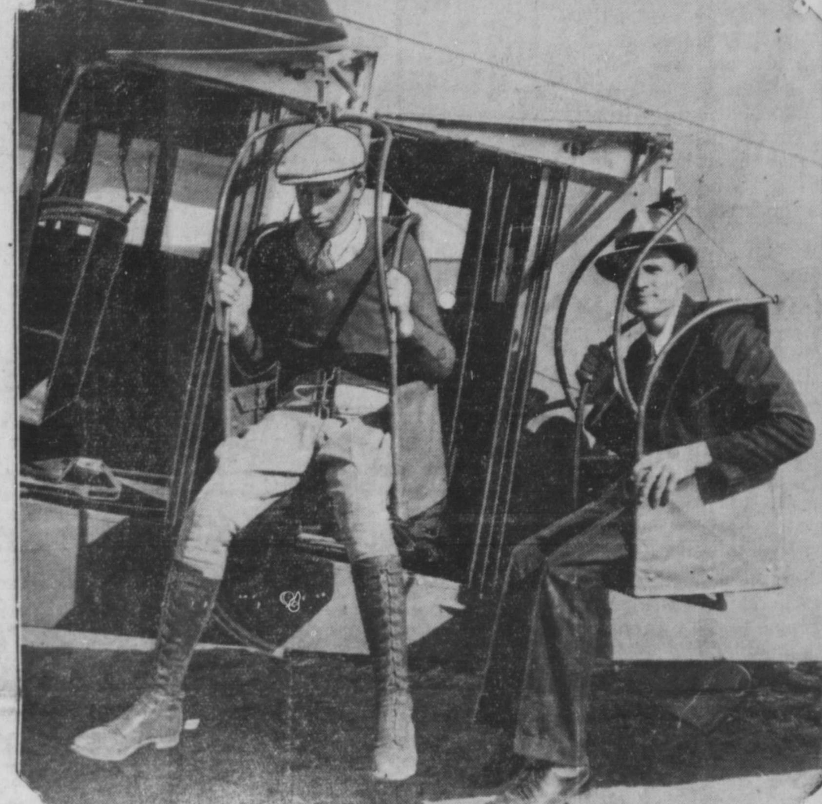
Swoosh! and down you go, whether you like it or not. Plane passengers, too nervous parchute jump in time of emergency, are automatically swung through separate doors and dropped by the pilot with this new apparatus tested in California.
