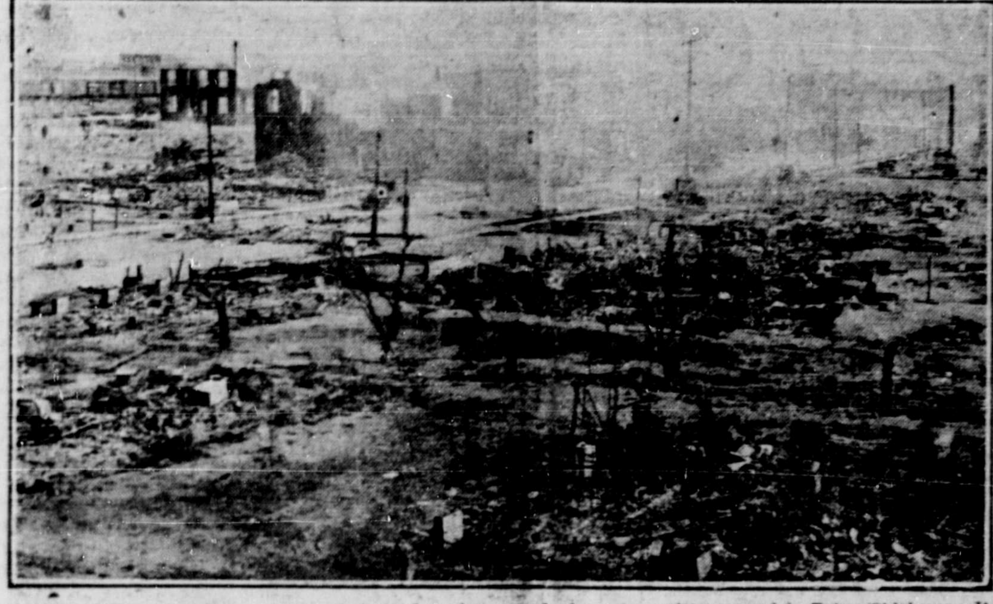
Ten blocks of negro quarters were burned to the ground when a race riot occurred in Tulsa, Oklahoma. It resulted in the death of 30 and the seriously injuring of several hundreds more. The photo shows part of the destruction wrought in the residential section.
