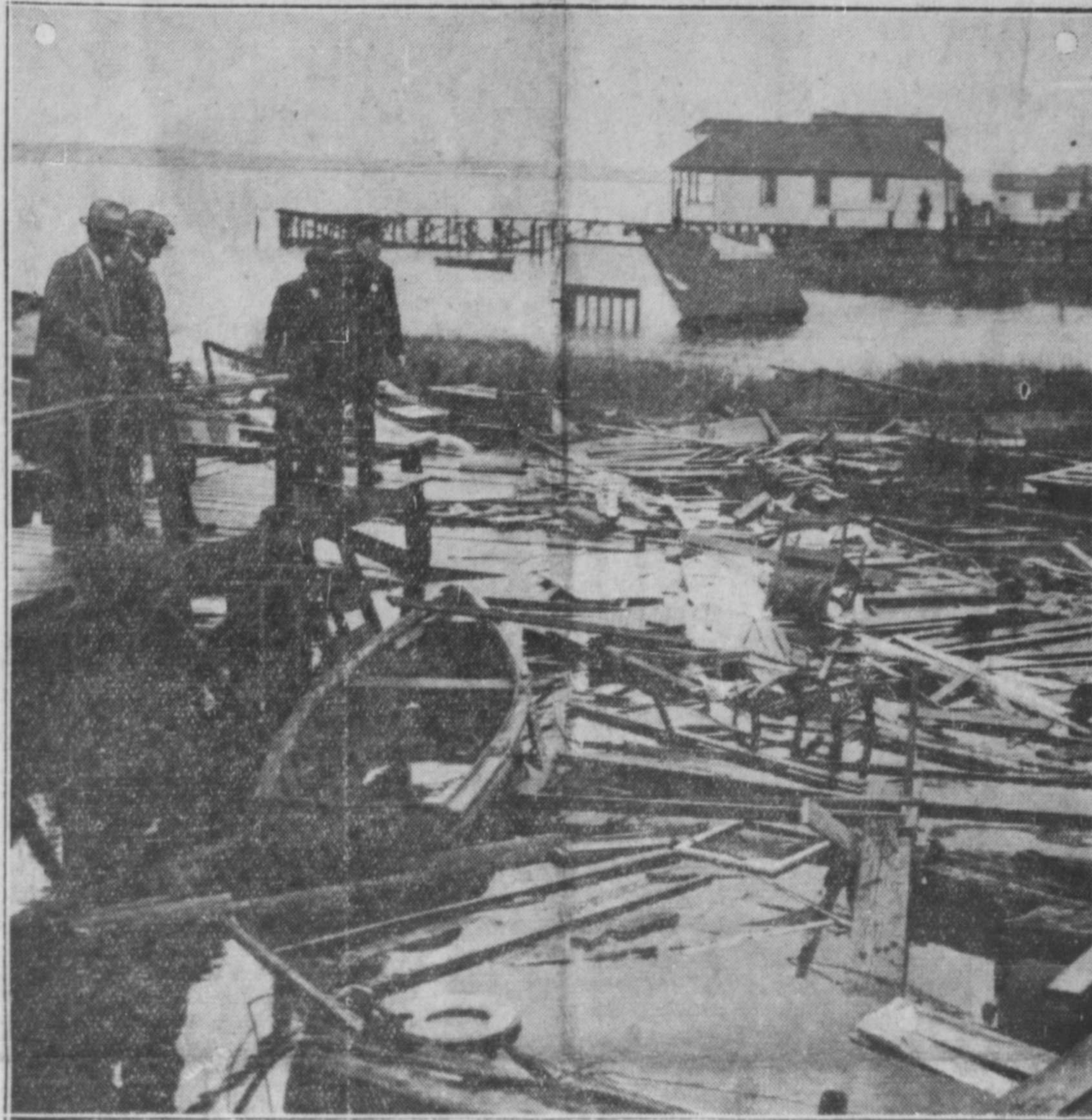
Twenty bungalows bungled into Jamaica Bay when a gale swept Long Island, N.Y., the other day. The wind, accompanied by a torrent of rain, succeeded in toppling over 60 others. The floating debris in the foreground was from a home.
