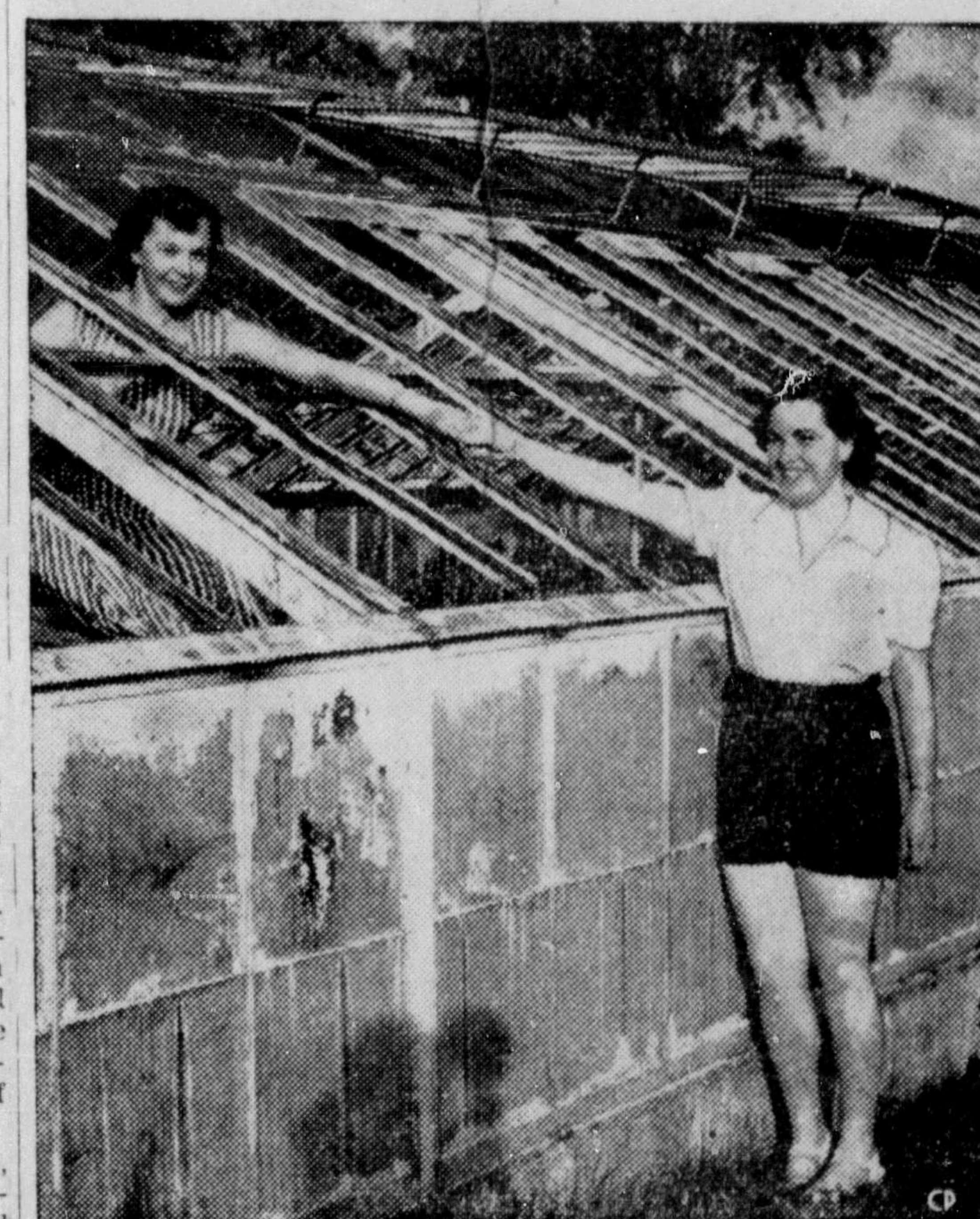
FREAK HAILSTORM —Two Ontario Agriculture department employees join hands through shattered frames in a greenhouse damaged when a freak hailstorm pounded the town of Kemptonville, Ont., 32 miles south of Ottawa. Estimates of damage to the town and surrounding area ranged from $100,000 to $500,000. Some of the hailstones were as large as baseballs. The greenhouse at the Kemptonville Agricultural college lost 1,700 panes of glass. (CP PHOTO)
