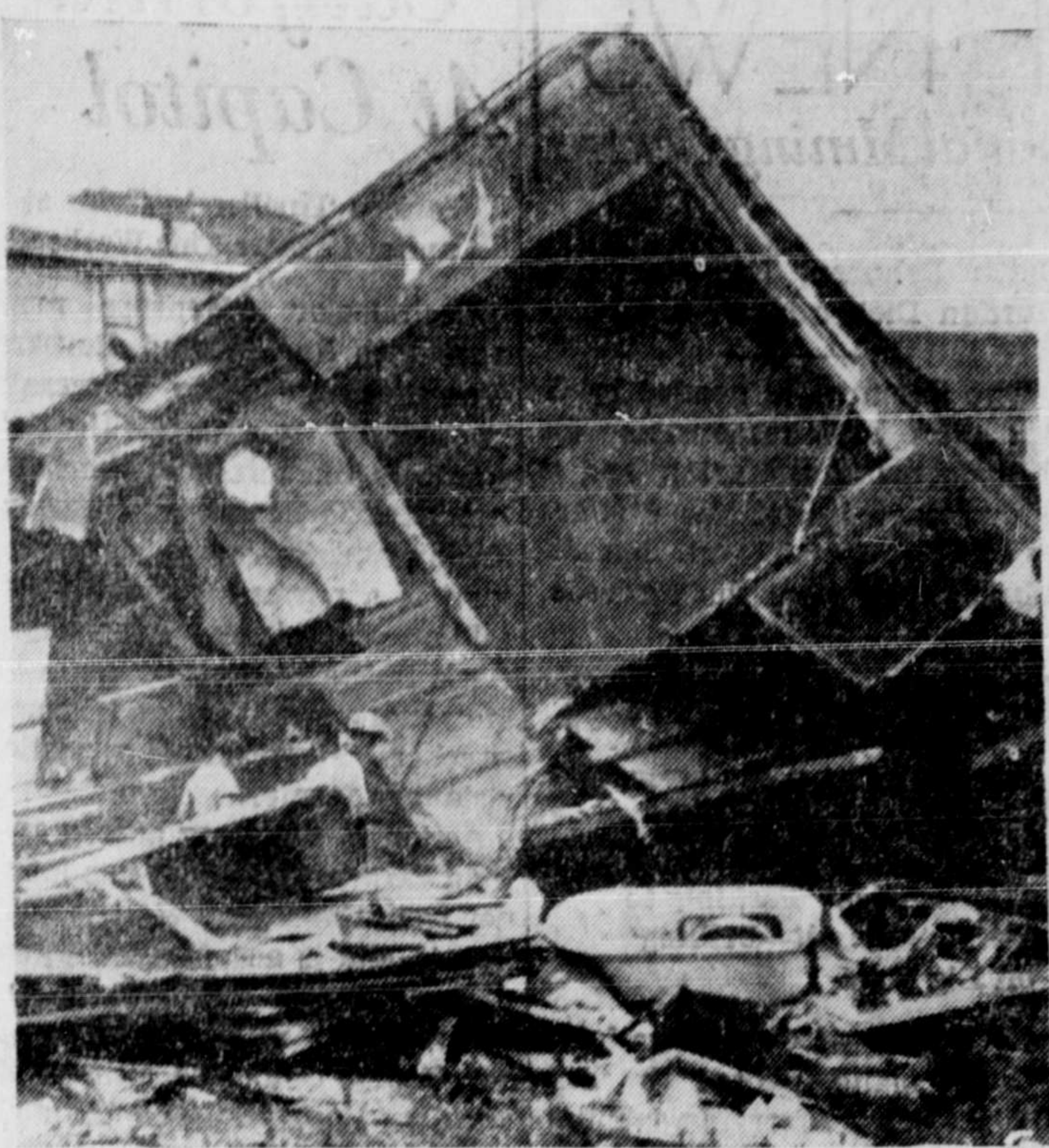
WRECKAGE LEFT IN TORNADO'S PATH —Wreckage is all that remains of a home in Sharon, Pa., after it was hit by a Tornado which swept through the town, killing six persons and injuring 150 others. More than 250 homes were damaged or destroyed. Telephone and power lines were destroyed and the street ruined over a large area.
