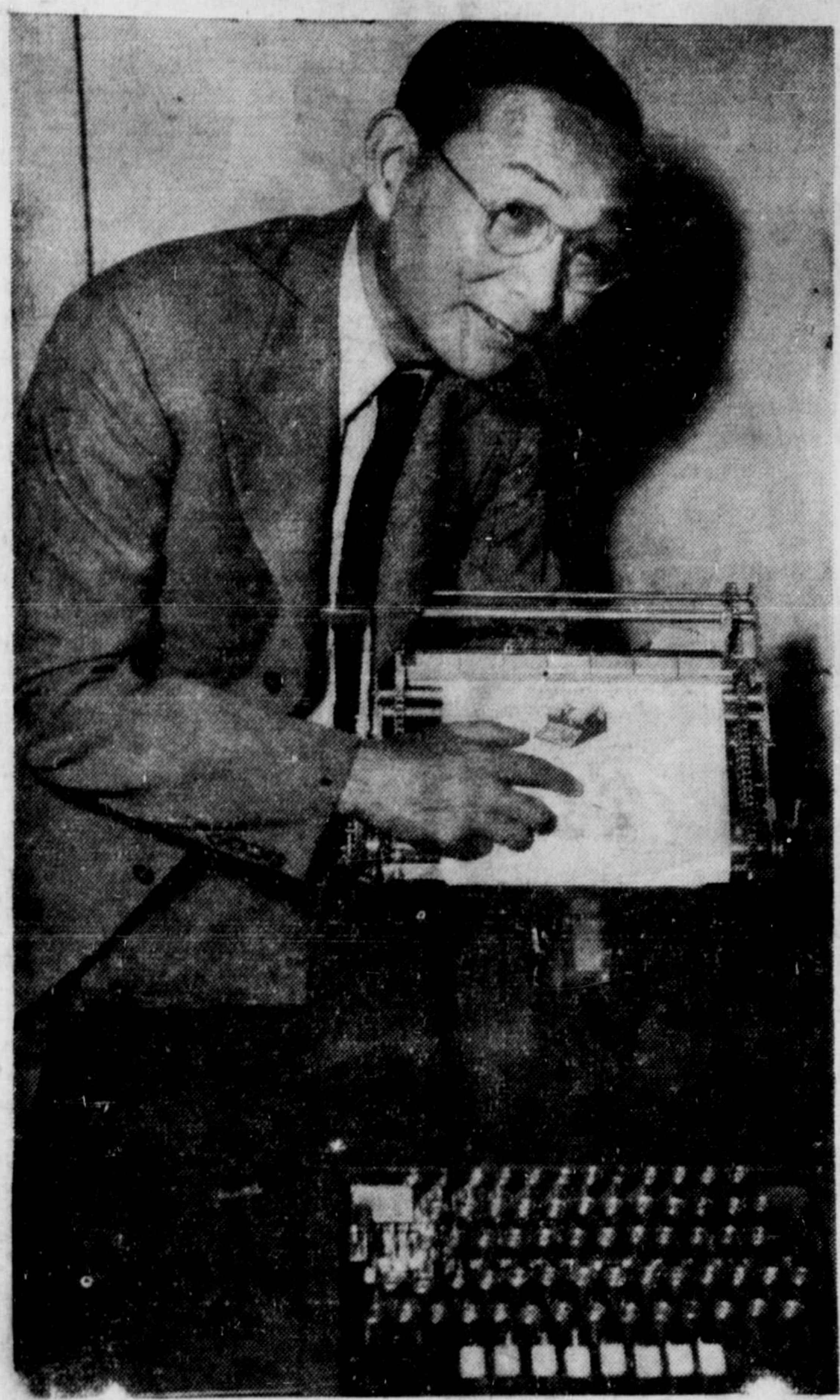
RAZING THE TOWER OF BABEL—Lin Yutang, Chinese author, is shown at his New York home introducing the Chinese typewriter, the fruit of 30 years' work, which he invented. It is the first Chinese typewriter which can type all known Chinese words. It can print 90,000 Chinese characters, requiring pressing of only three keys for each word. In addition it can type English, Japanese, Russian and the Chinese phonetic alphabet. With it, a typist can do in an hour the work of a Chinese copyist for a day. Lin Yutang's invention is the only Chinese typewriter which requires no previous training to operate. It is no larger than the standard American machine.
