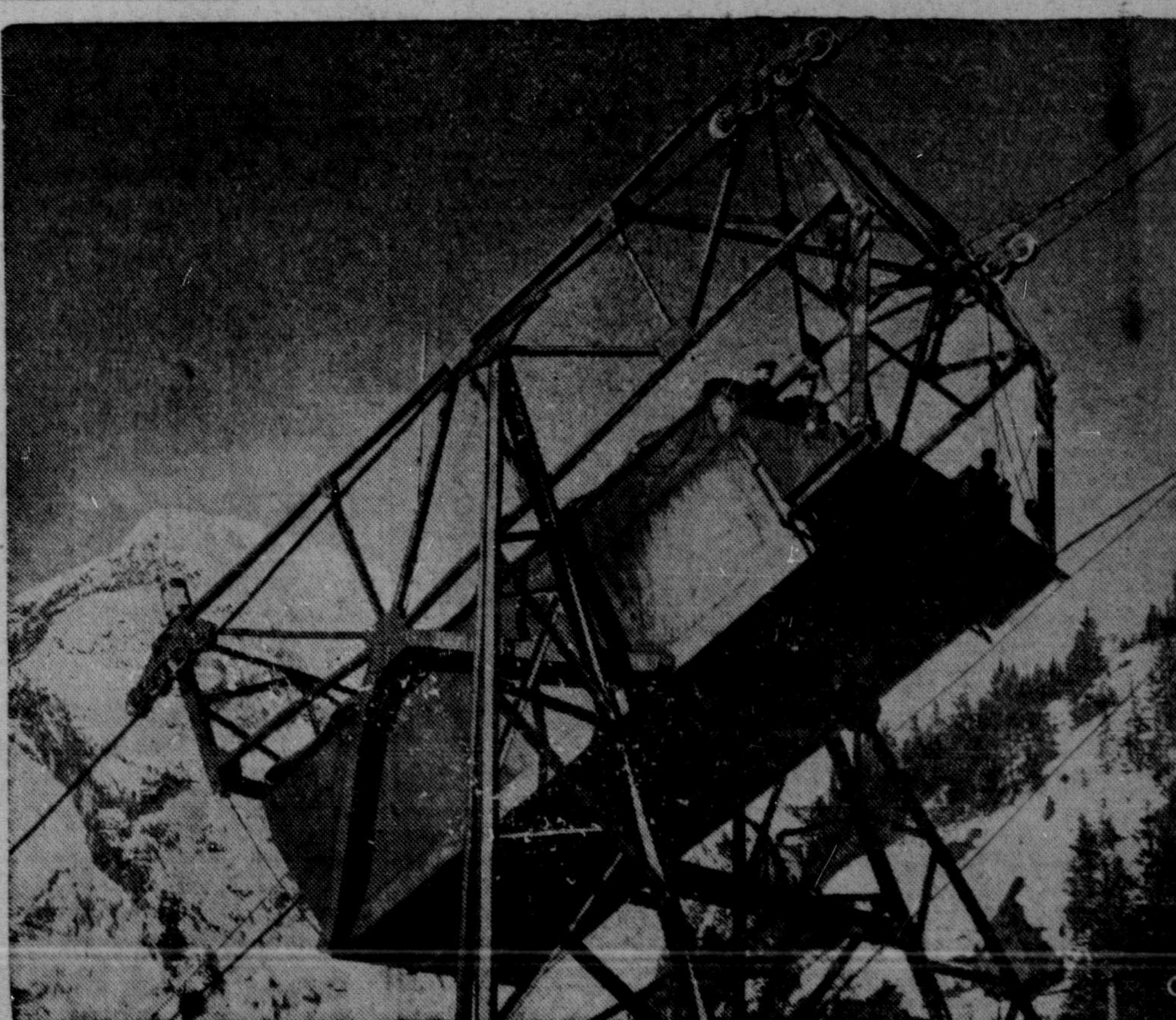
MEN AND MACHINES are tunnelling 10 miles through a mountain to provide cheap power for British Columbia's new aluminum industry. Deep inside the mountain, 1,400 feet underground, a bomb-proof, weather-proof powerhouse for the Aluminum Company of Canada is being scooped out. Some of the tunnelling is done from the 1,600- and 2,600-foot levels of the mountain. These camps are served by cable tramline which creeps up an incline averaging 30 degrees with a 20-ton load on its back. (CP PHOTO)
