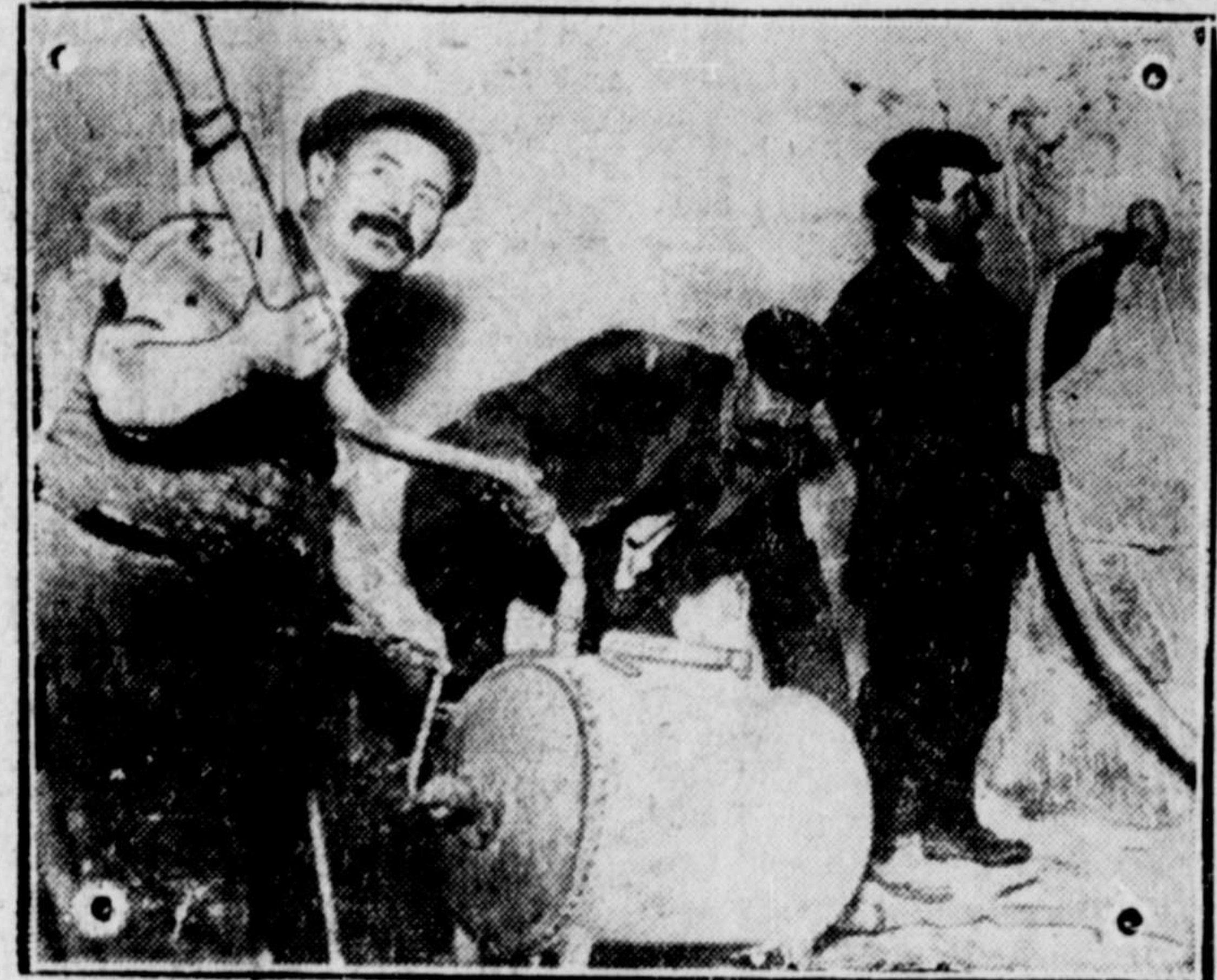
Workmen are filling the cracks in the dome of the new St. Paul's Cathedral, London, with compressed cement in their effort to save the towering edifice that has overlooked the city for so many years.
