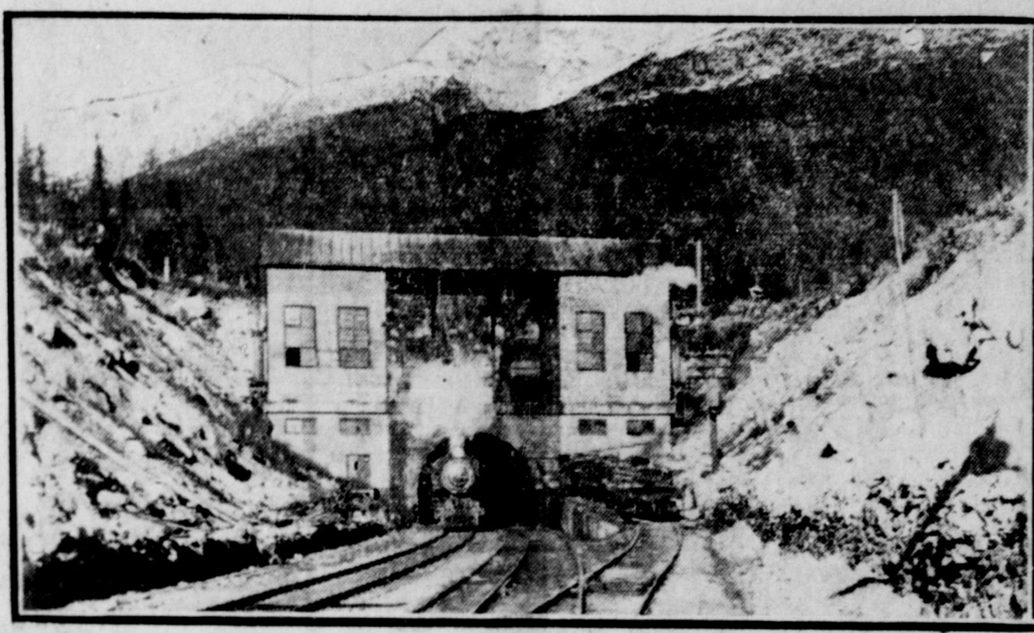
Connaught tunnel, five miles long, near Field, B.C. Its construction constitutes an engineering epic. Starting at both ends the engineers bored through solid rock to meet exactly.
