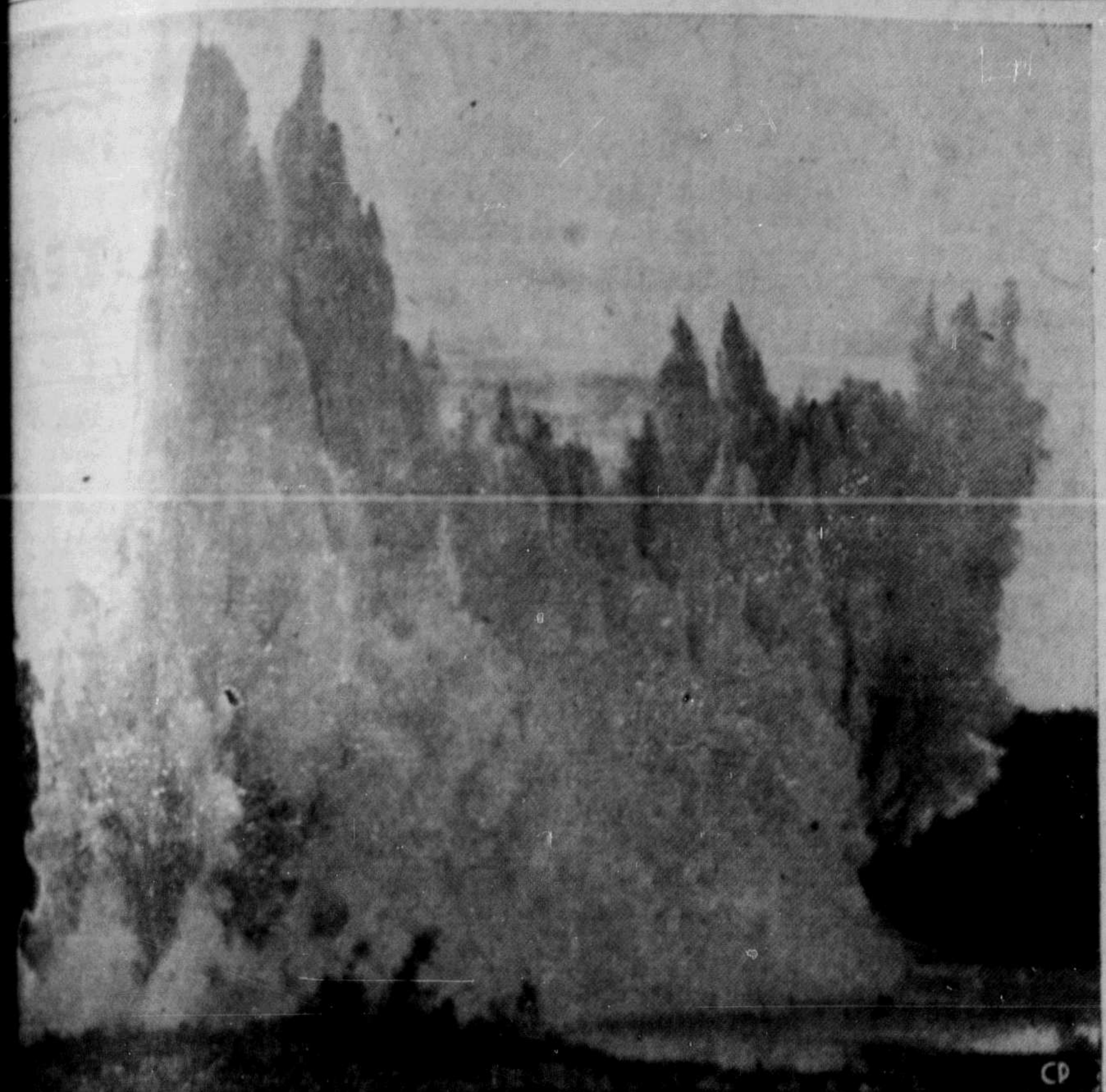
PATTERN—A 6½-ton dynamite blast makes an unusual pattern throwing more than tons of rock, mud and Rideau River water into the air. The blast, a few miles southeast of here, made a trench in the river bottom for one of the last sections of the Trans-Canada Pipe Line Company's 440-mile linking Hamilton, Ottawa and Montreal. The line carries gasoline, diesel oil and domestic and fuel oil. (CP PHOTO)
