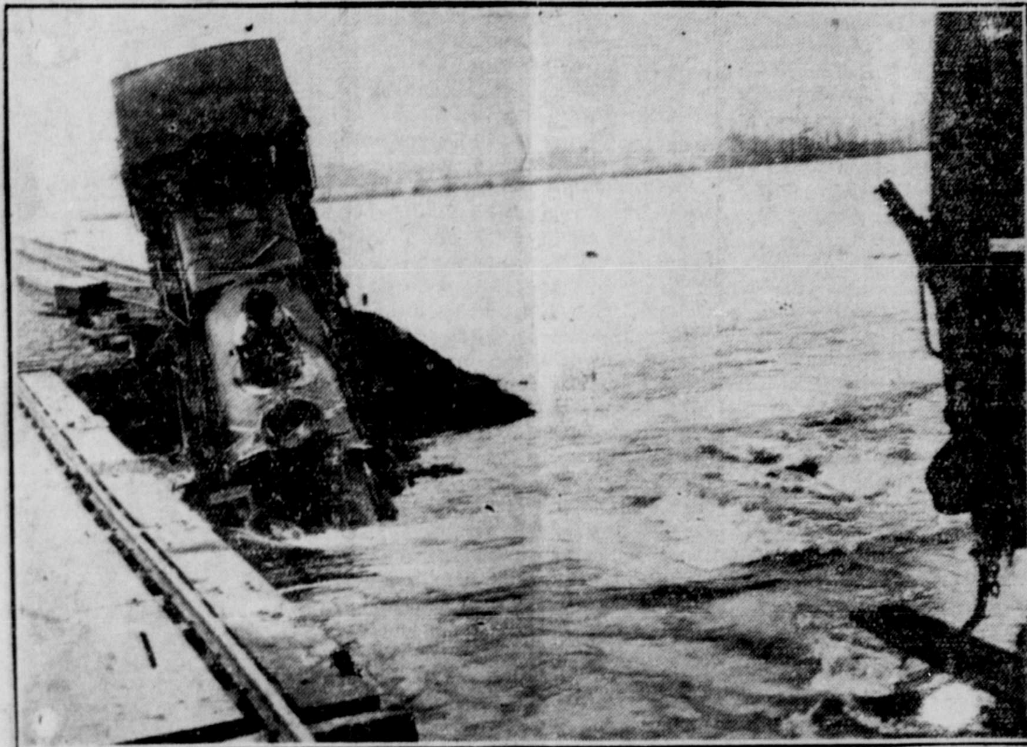
DYKE BREAK CAUSES TRAIN WRECK—The above graphic photo illustrates one of the terrible results of the breaking of a dyke near Beugen, Holland. The tracks were washed away and the speeding train was derailed into the water. Floods in Holland are said to have caused more damage than any other similar disaster in years.
