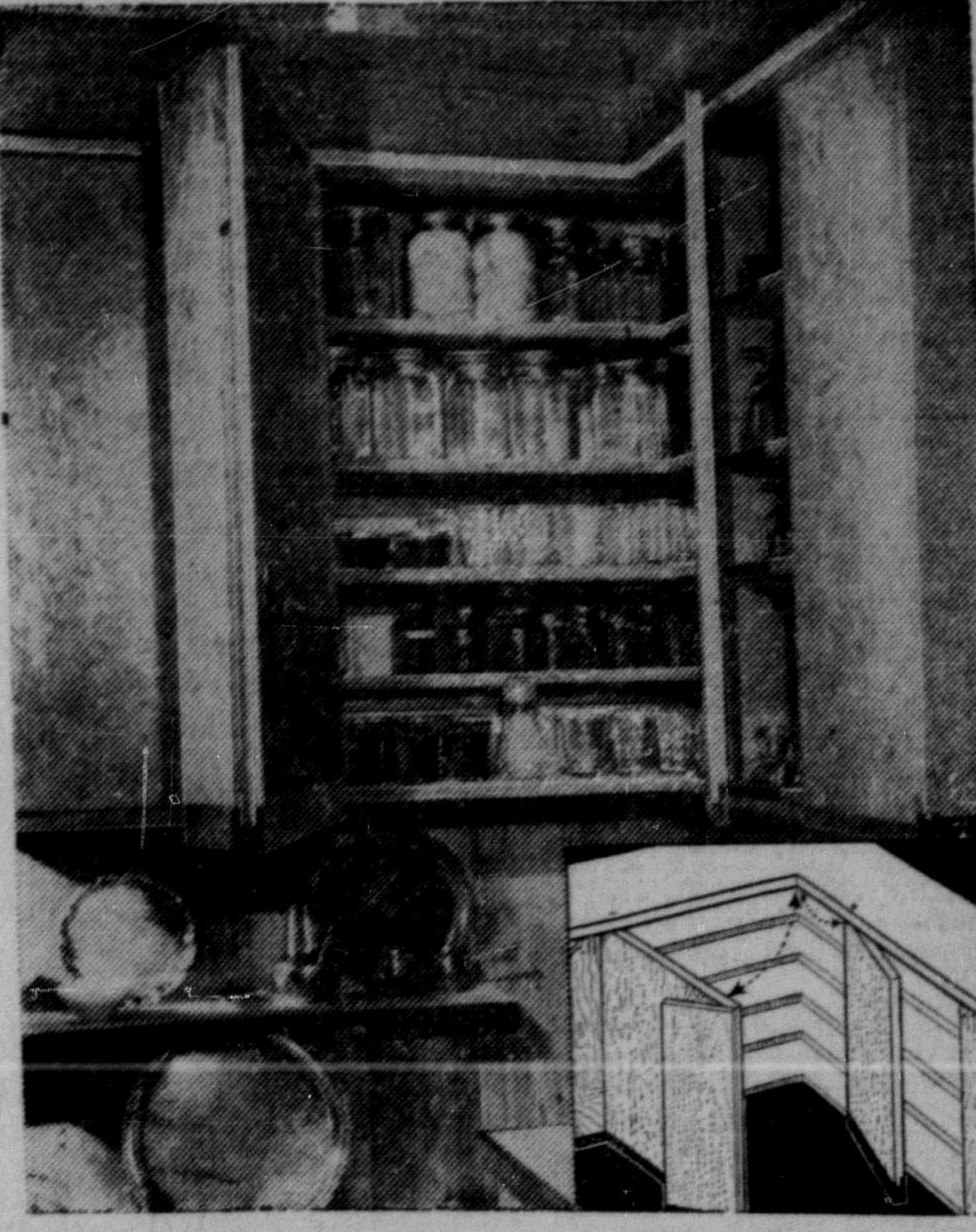
HARD TO GET AT CORNERS in kitchen cupboards can be eliminated. One idea shown here features a double-hinged door of plywood. The partition between cupboards is offset from the corner leaving that area completely accessible. Plywood corner cupboards like these can be built at home or easily put in by your carpenter.
