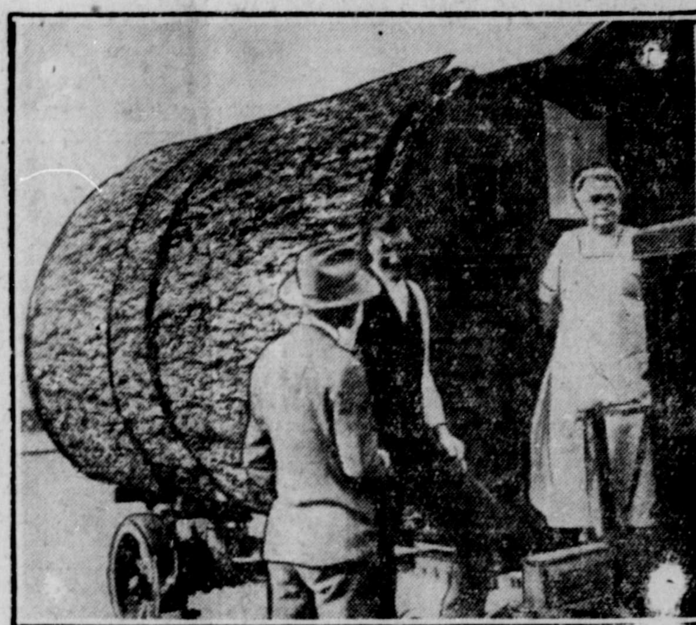
MR. AND MRS. E. A. WADE made a house of a Douglas fir log, 9 feet 4 inches high, and mounted on a truck and trailer. It is 16 feet long and divided into two rooms. The tree started to grow in 1492, and when cut was 311 feet high, containing 50,000 board feet of lumber
