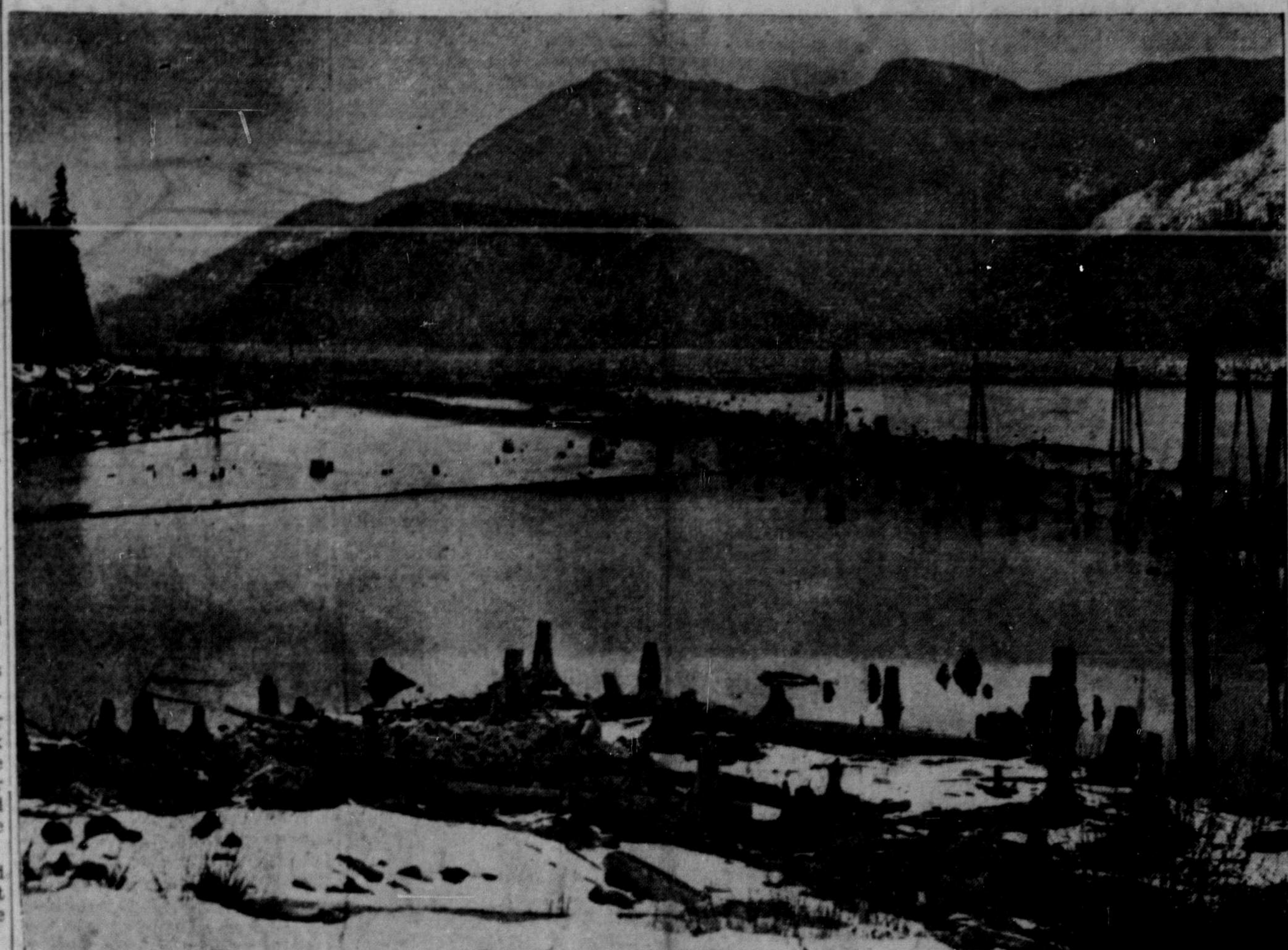
A MONUMENT OF SNAGS —This photograph shows what happens when an area is flooded for the purpose of producing hydro electric power without the removal of trees from the projected shoreline of such a lake. Stave Lake was flooded by building of the Ruskin Dam in 1920 to produce power for the B. C. Electric Company. Today, the dead snags still present an eyesore along the entire perimeter of the lake which
