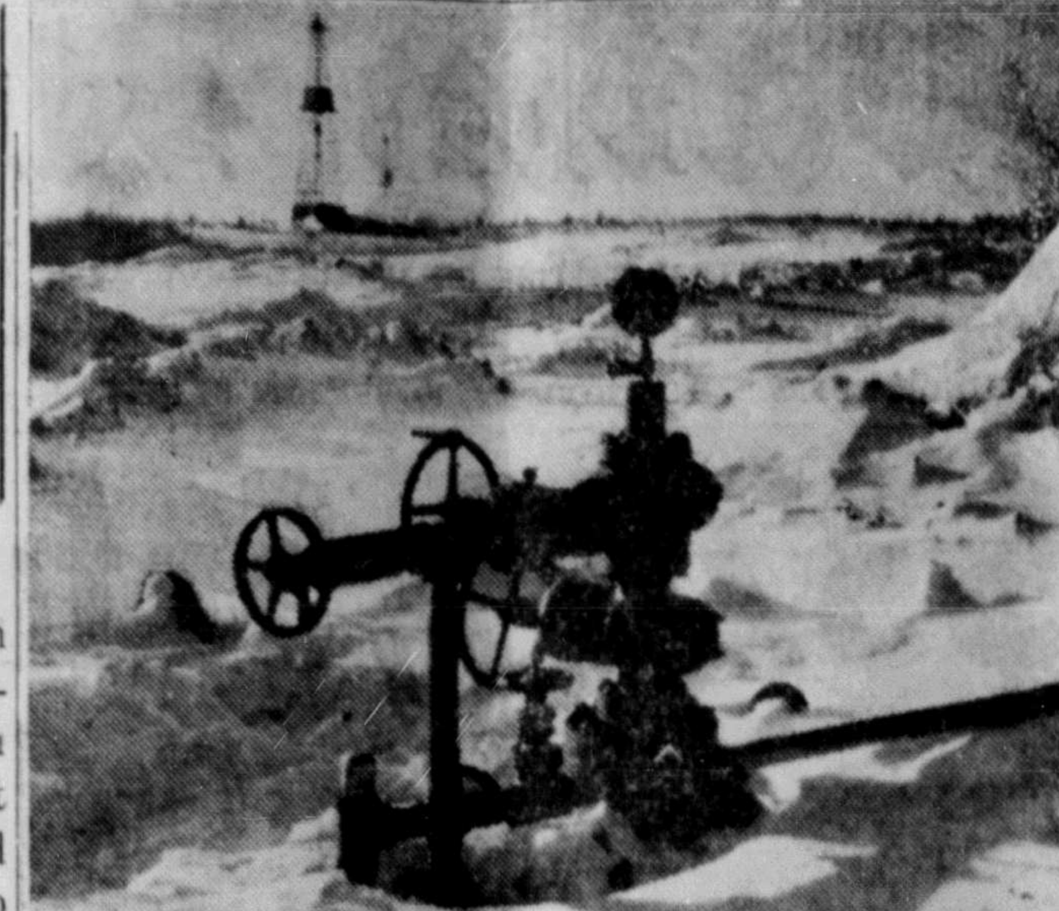
WINTER AT LEDUC—Drilling continues in summer and winter in Alberta's flourishing Leduc oil field. While one well is already producing oil (foreground) the tall derricks in the background shows where further drilling is being carried on. The pipes, wheels and valves of the producer are called "Christmas trees." (CP PHOTO)
