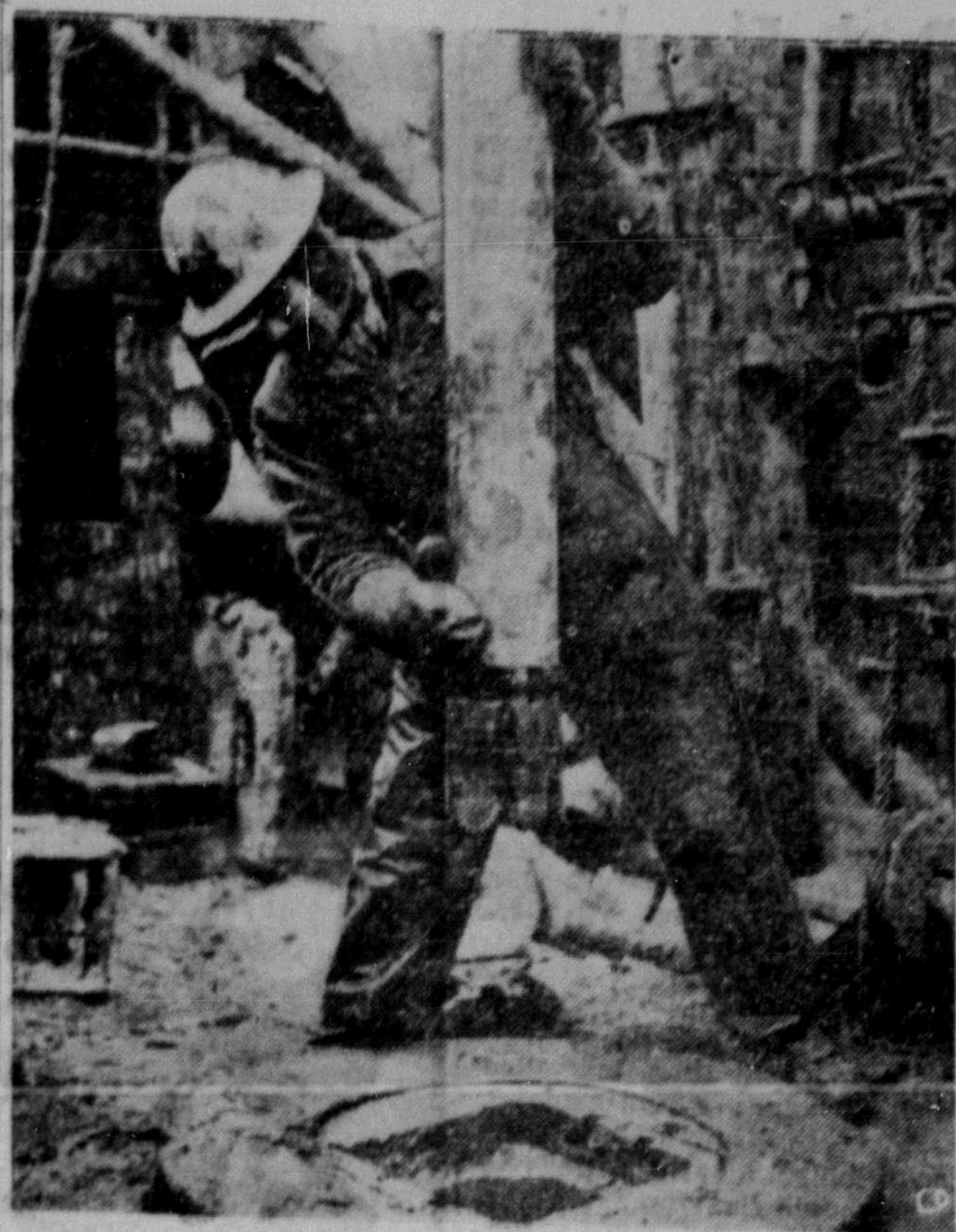
MODERN DRILL —A driller at one of Imperial Oil's extension wells in the Leduc-Woodbend area of Alberta guides the drill stem and bit into the rotary table after changing a drilling bit. Boring through hard rock galls even the tough metal of the bits which must be changed frequently. (CP Photo)
