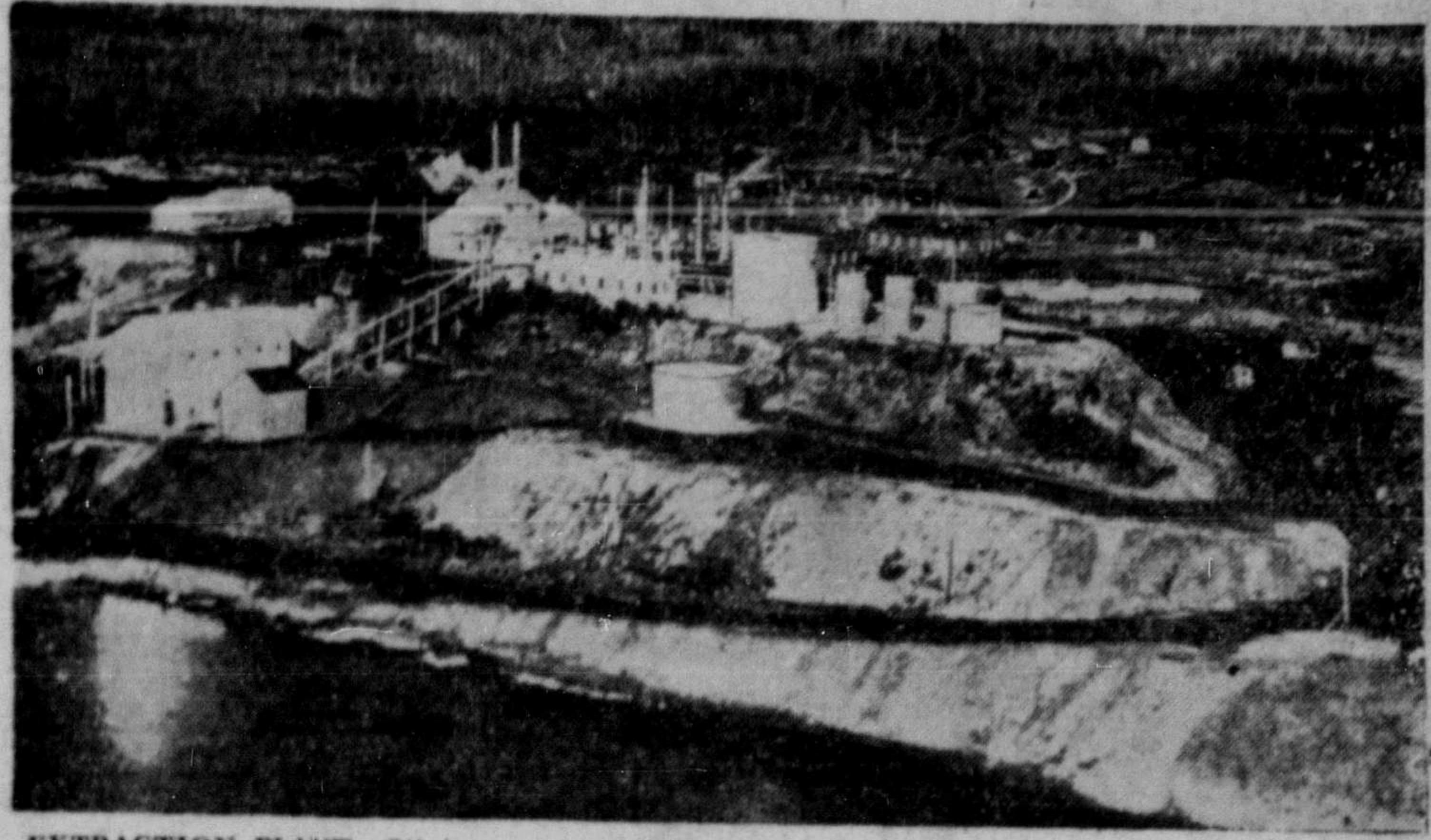
EXTRACTION PLANT —Oil is extracted from Alberta's oil sands in this provincial government plant at Bitumont on the Athabasca river. The extraction method includes the use of hot water and steam. Swedish interests will use part of the plant for experiments with another extraction method. In this photo the sand outcrop on the Athabasca river is shown. At lower right is the quarry from which sand is taken for the pilot plant operation.
