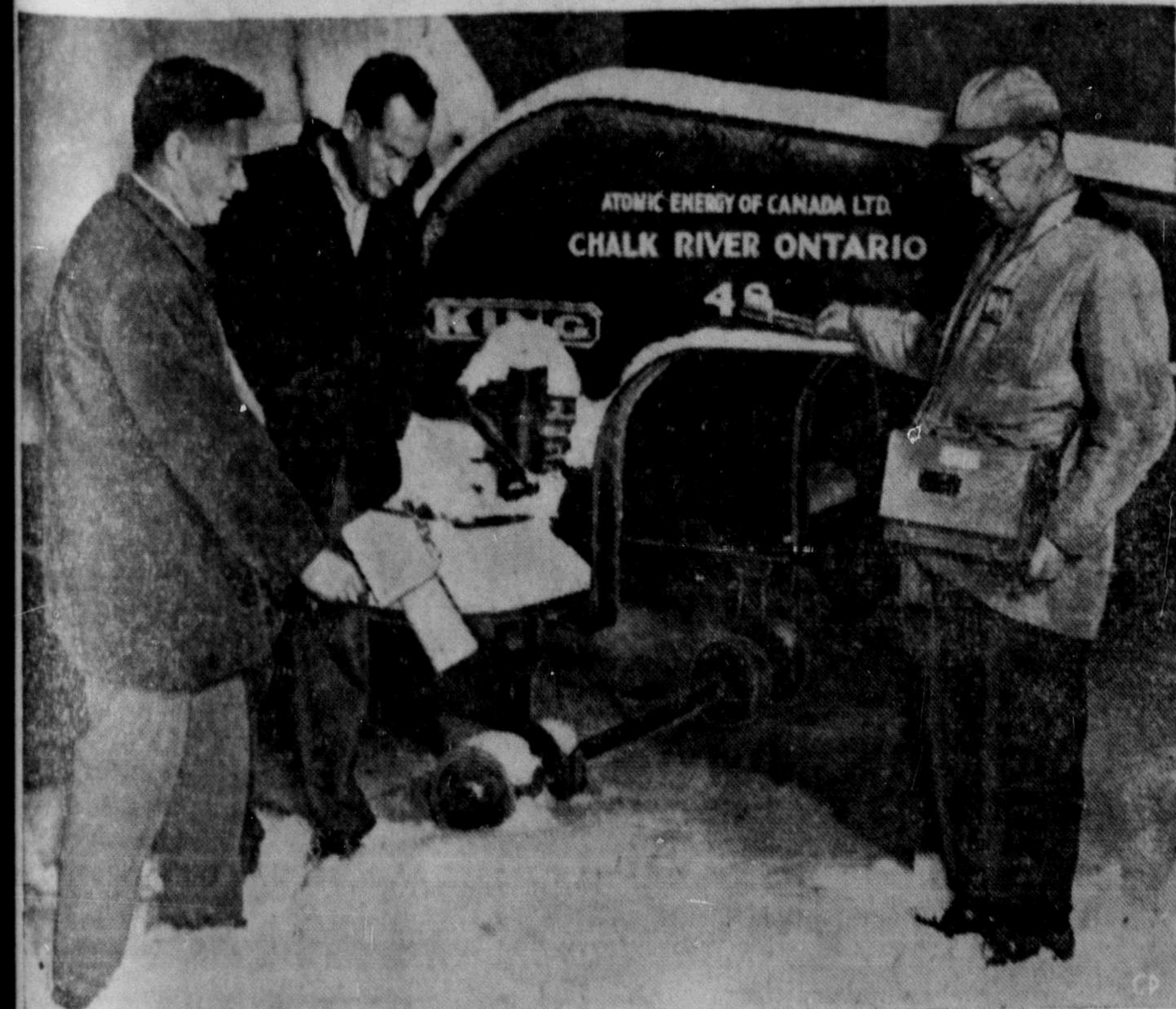
DECONTAMINATION SQUAD at the Chalk River atomic plant explores the area with geiger probes and a radiation survey meter are shown checking for excessive radiation which leaked through a pin-point hole in the big atomic pile last week and forced evacuation of the 350 workers. Left to right are: Campbell Tait, head of the radiation hazard control branch; Dr. A. L. Cipriani, director of the division of biology and radiation hazard control, and Charles L. Cleveland, radiation supervisor.
