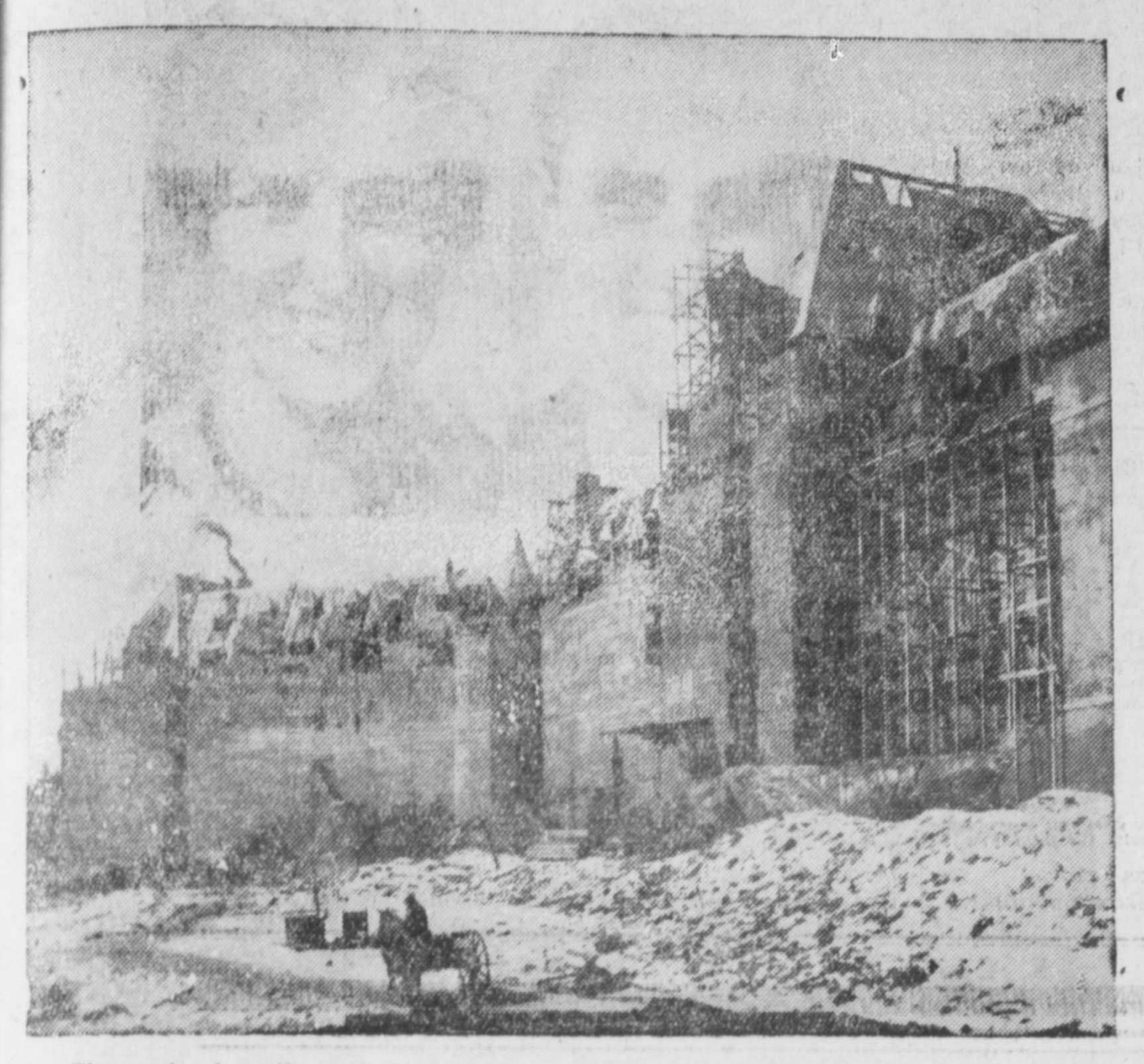
The work of peeling off the wooden shell under which the new Manoir Richelieu has been building all winter, was begun last week. The glazing of windows on the first two floors is now in progress and the gleaming copper roof is in place. The picture above shows the towers and part of the walls emerging from the encasing structure.
