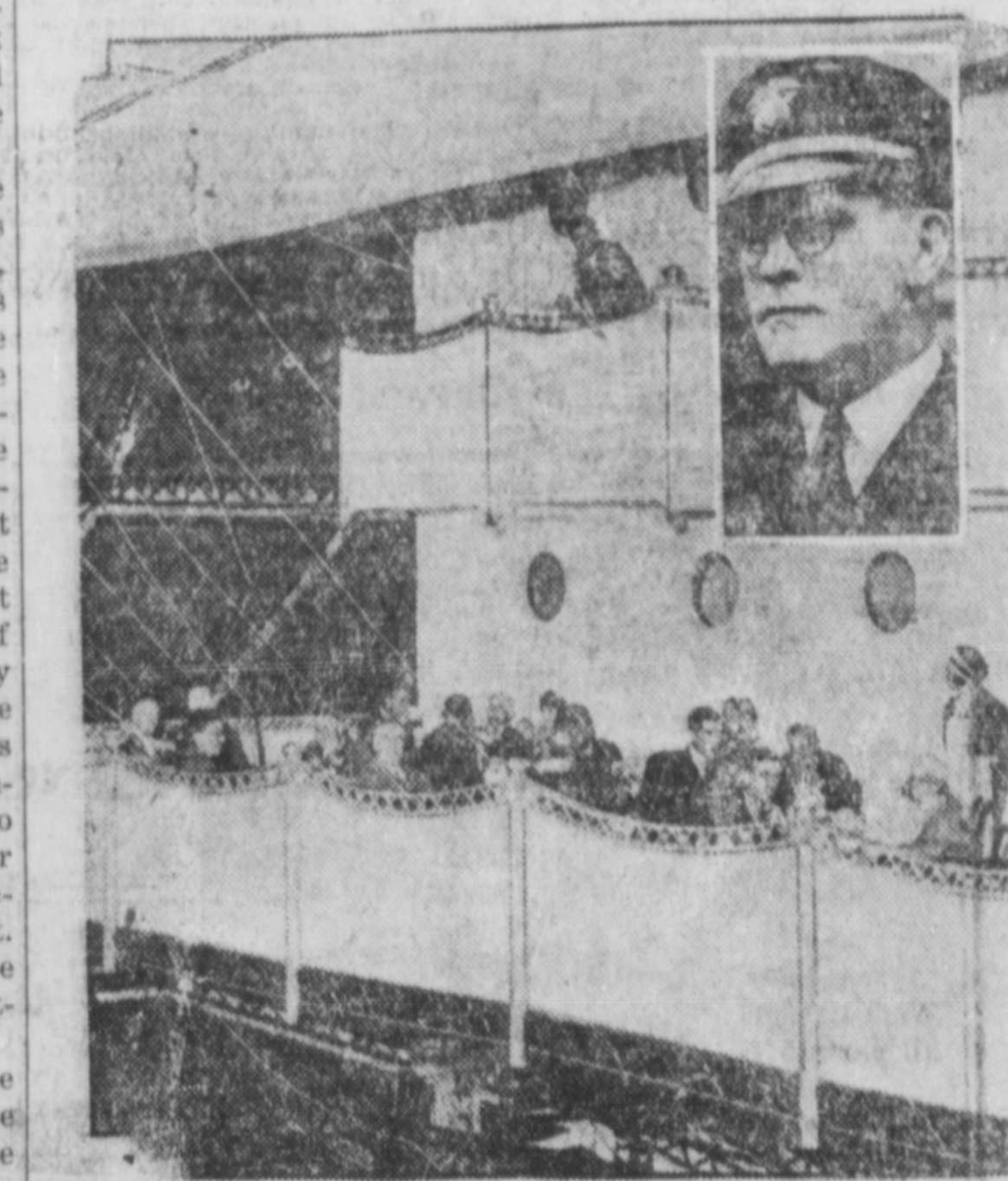
The amazing British airship, R-100, is at present undergoing tests at Howden, England, preparatory to flying to Canada in the spring. This giant dirigible is 709 feet long, 130 feet high, and will easily carry 135 passengers, inclusive of crew. Six Rolls Royce engines will drive her through the air at a cruising speed of 75 miles an hour, and she is expected to complete the ocean flight in less than three days. The above picture shows members of the Mother Parliament having tea aboard the R-100 at her formal unveiling to the public. Inset is Lieutenant George Norville, who will navigate the giant air liner on her maiden voyage.
