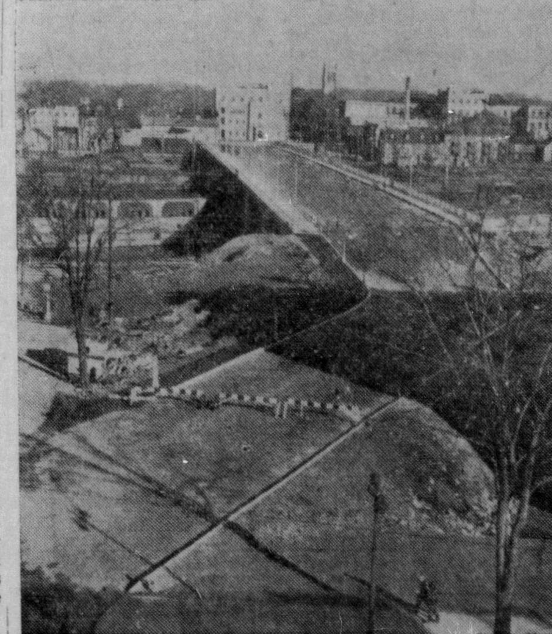
OTTAWA'S NEW BRIDGE—The new Mackenzie King bridge, first major project in Ottawa's beautification plan, will be opened to traffic shortly. This photo shows the temporary approach which links the bridge with Albert Street. Casting a shadow across the approach is the Aymer Building which is to be removed in the spring to make way for construction of a similar connecting link with the bridge at Slater Street, across the Rideau canal. When completed it will serve as a route through the National capital and help relieve traffic on Confederation Square, often referred to as "Confusion Square." (CP Photo)
