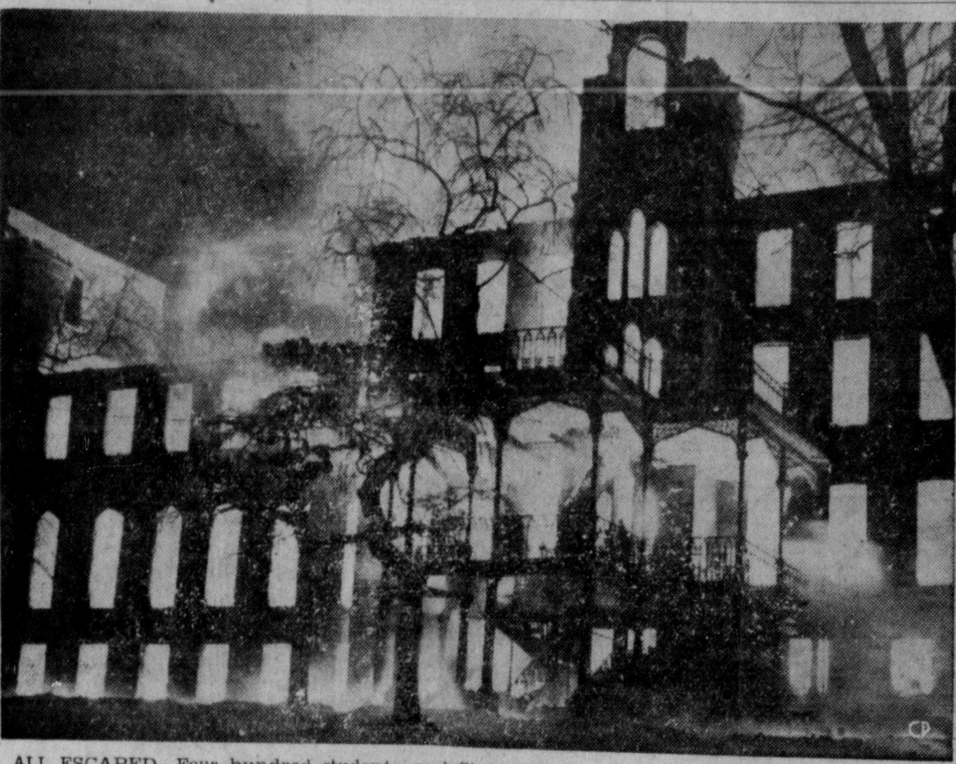
ALL ESCAPED—Four hundred students and Sisters of Charity escaped without injury when fire destroyed the main building of Mount St. Vincent College near Halifax. Twice-weekly fire drills paid off as students filed out in what many believed to be just another practice. (CP PHOTO)
