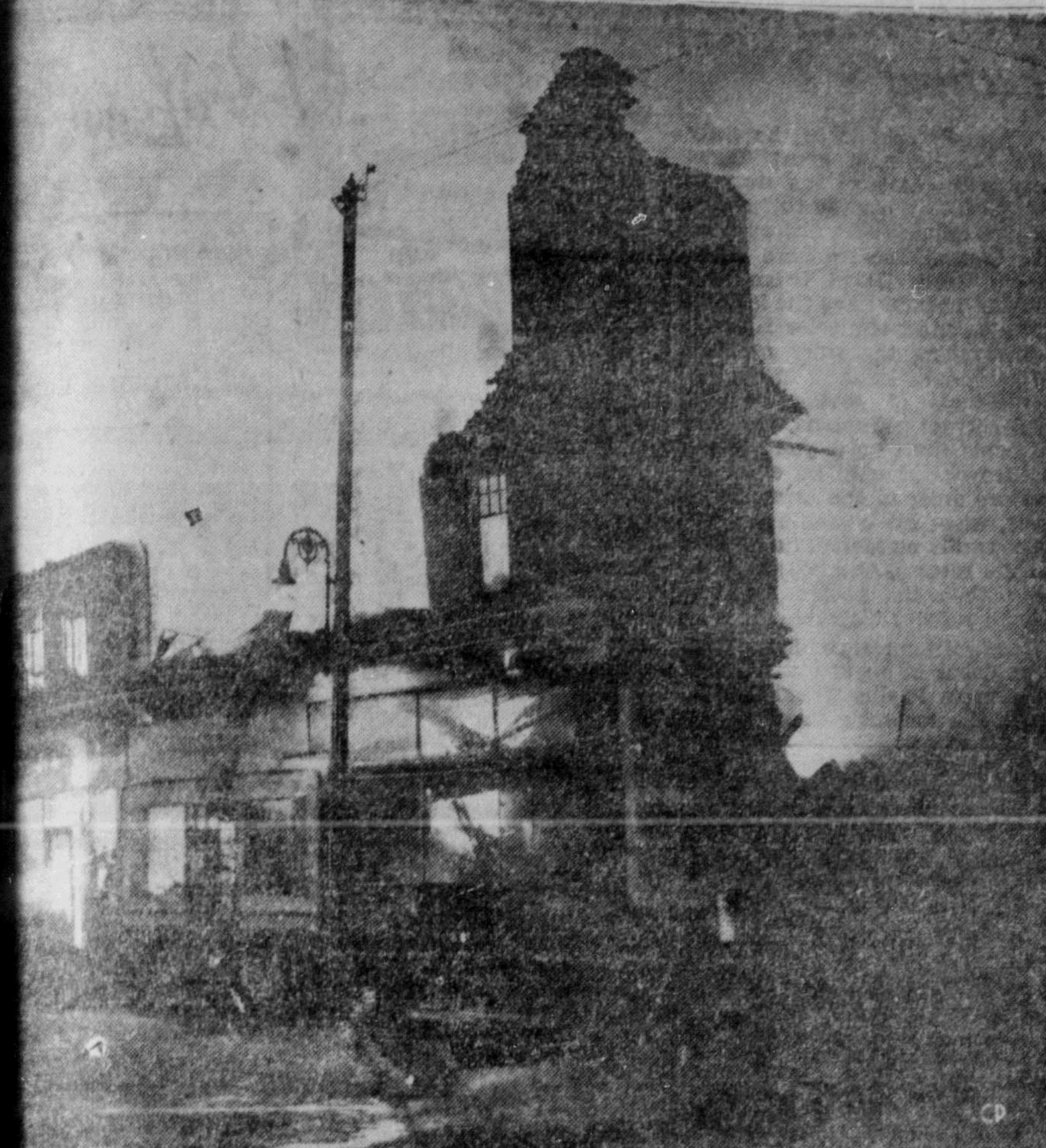
HOTEL BURNS —Two walls have fallen showing fire still raging through the ruins of the Hotel Burns at St. Thomas, Ont., which was destroyed by fire early Sunday morning. One man is believed to have perished in the fire. This graphic photo shows one corner of the hotel still standing. Damage was estimated at $300,000. (CP Photo)
