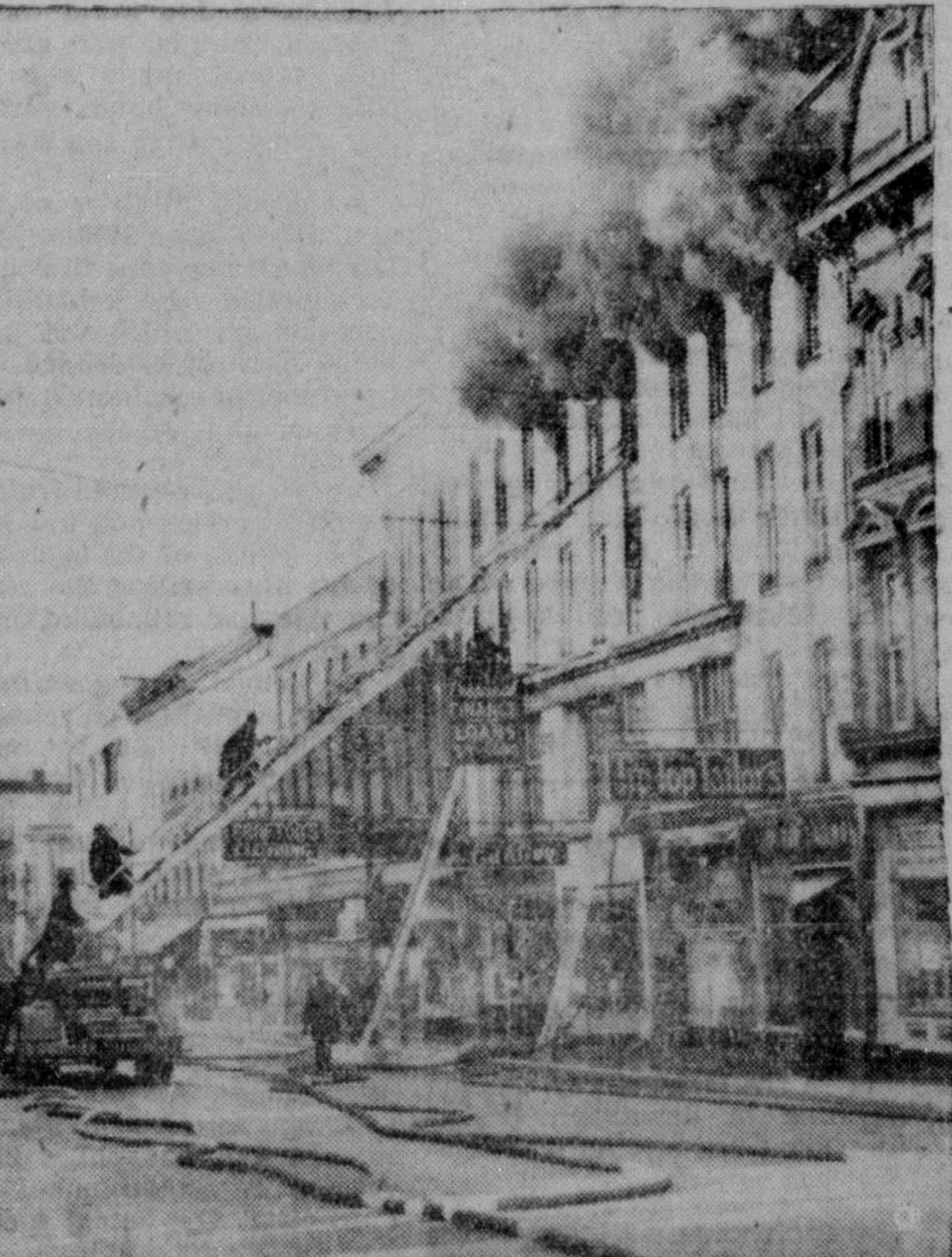
FOUR DIE IN FIRE —Three firemen and a volunteer were killed in this fire at Peterborough, Ont., when ceiling and floors collapsed. The building—in the centre of the city's business district—was a total loss. Damage was estimated at $300,000. (CP PHOTO)
