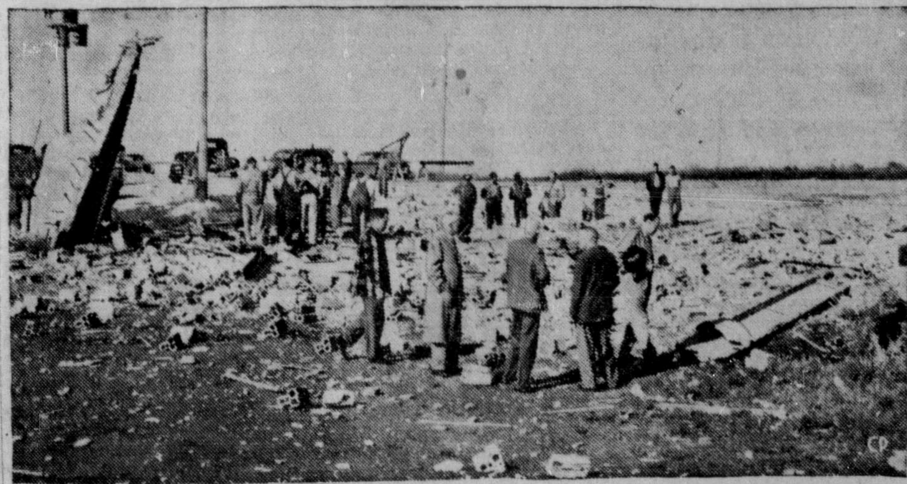
BLAST IN SASKATOON—Saskatoon's three-year-old sewage disposal plant was razed by a violent explosion, believed to have been caused by gasoline leaking into the sewers. No one was hurt in the blast, which caused an estimated $100,000 damage. (CP PHOTO)
