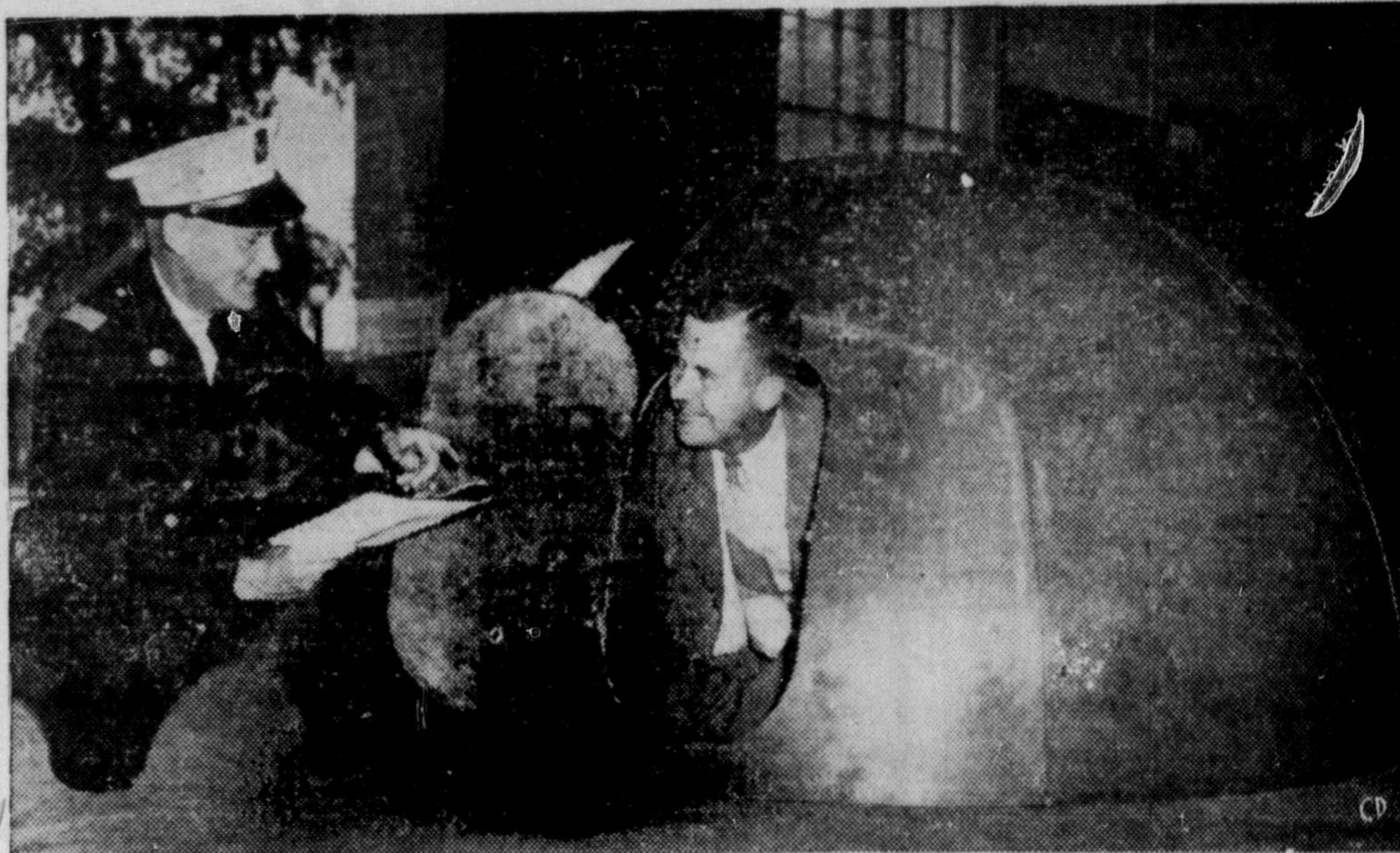
NEW BOMB SHELTER —D. E. Auten, right, development engineer of the Firestone Rubber Co., shows off the company's new prefabricated, igloo-like bomb shelter to Fire Chief Earl Becker of Ottawa, during a display in the capital. Suitable for backyard use, the hemispherical unit comes in readily-assembled interchangeable sections and is designed for use over an excavation with a fourfoot fill of earth over it. It is reached by tunnel from a basement or subway ramp. (CP PHOTO)
