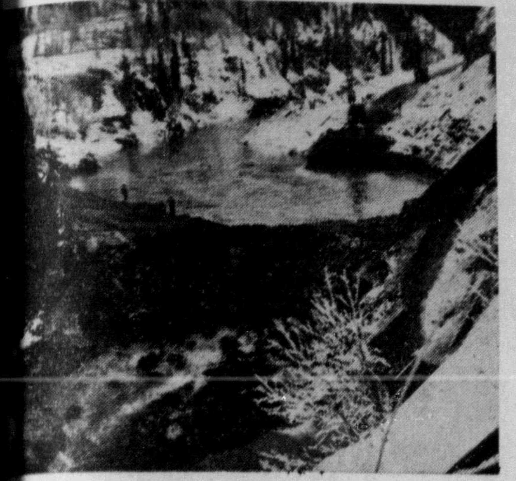
MAKO DIVERSION—Here is shown the cofferdam which was in connection with the diversion of the waters of the Nechako far in the interior south of Vanderhoof, into the western Kootenay River which will supply the Kitimat aluminum smelter.
