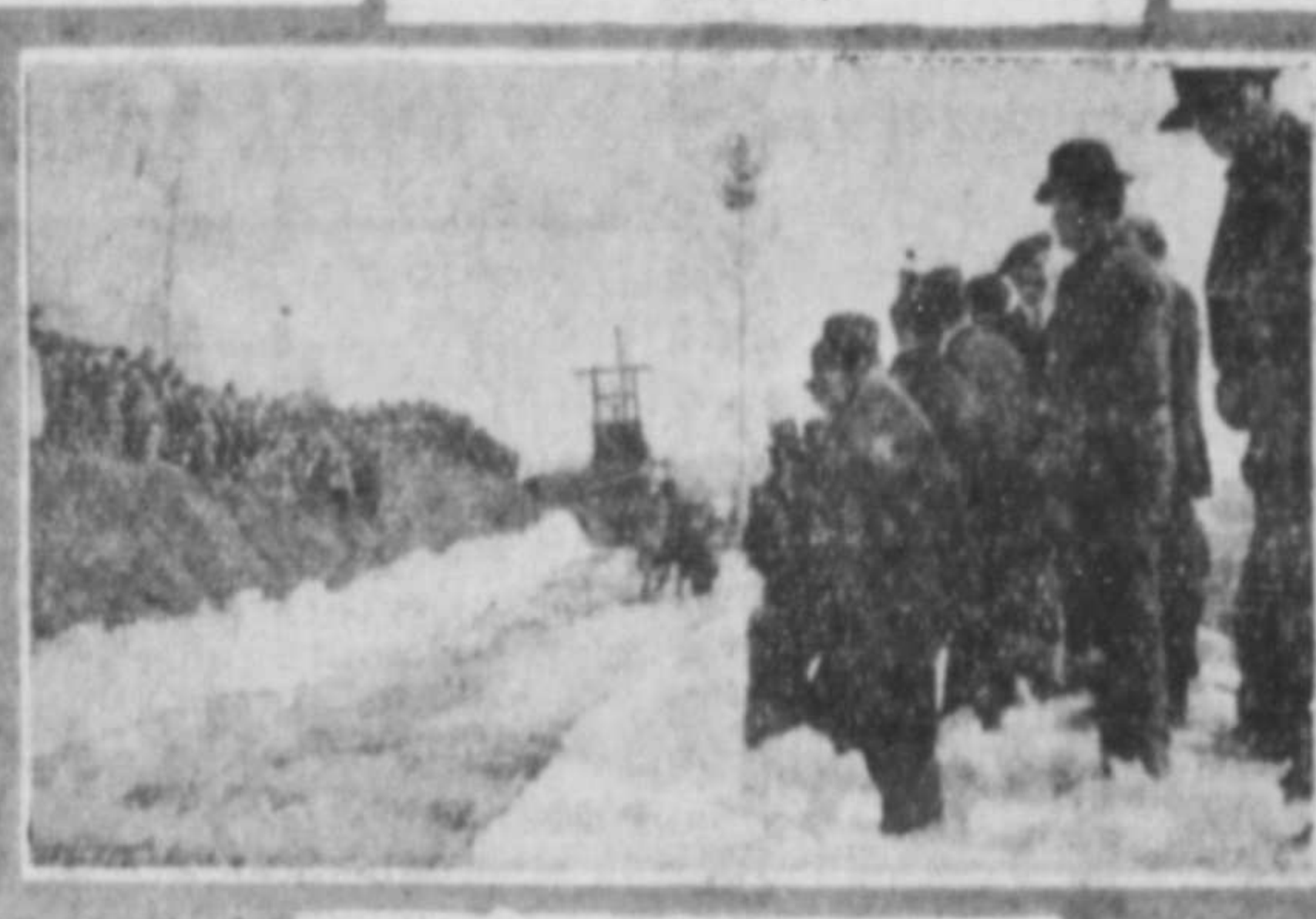
Track-layers making the last connection on the G.T.P. on Apr. 7, 1914, near Ft. Fraser
