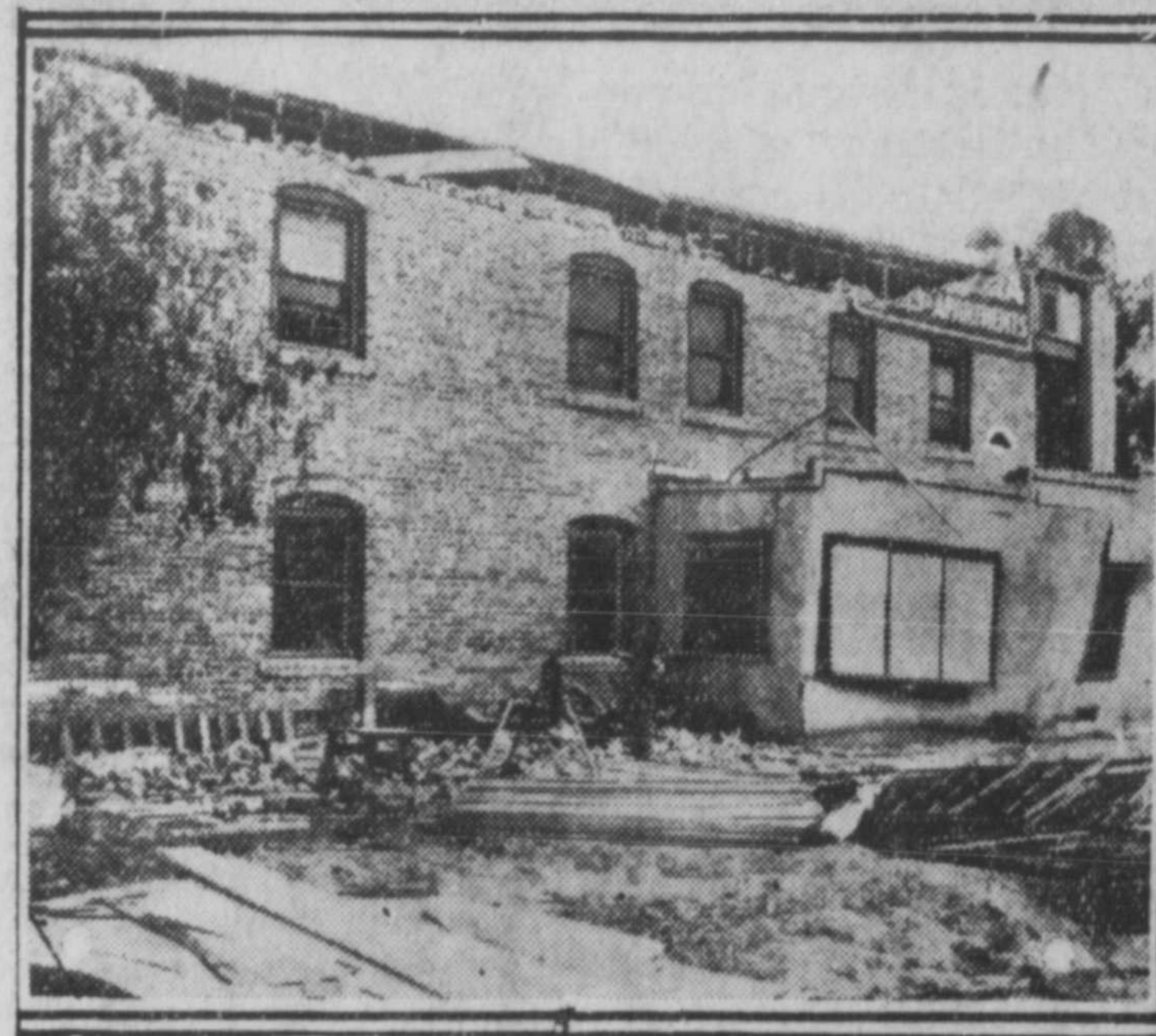
Sample of work done by recent earthquakes in Southern California. This apartment house in Brawley, Cal., in the Imperial Valley, was rocked and many bricks loosened from its structure.
