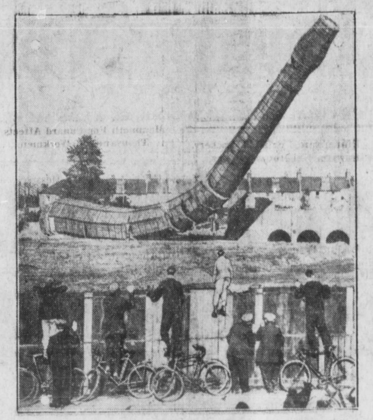
This 150-foot chimney at Tootin . England, is seen toppling with its 800 tons of brick just after a blast shook it from its base,
