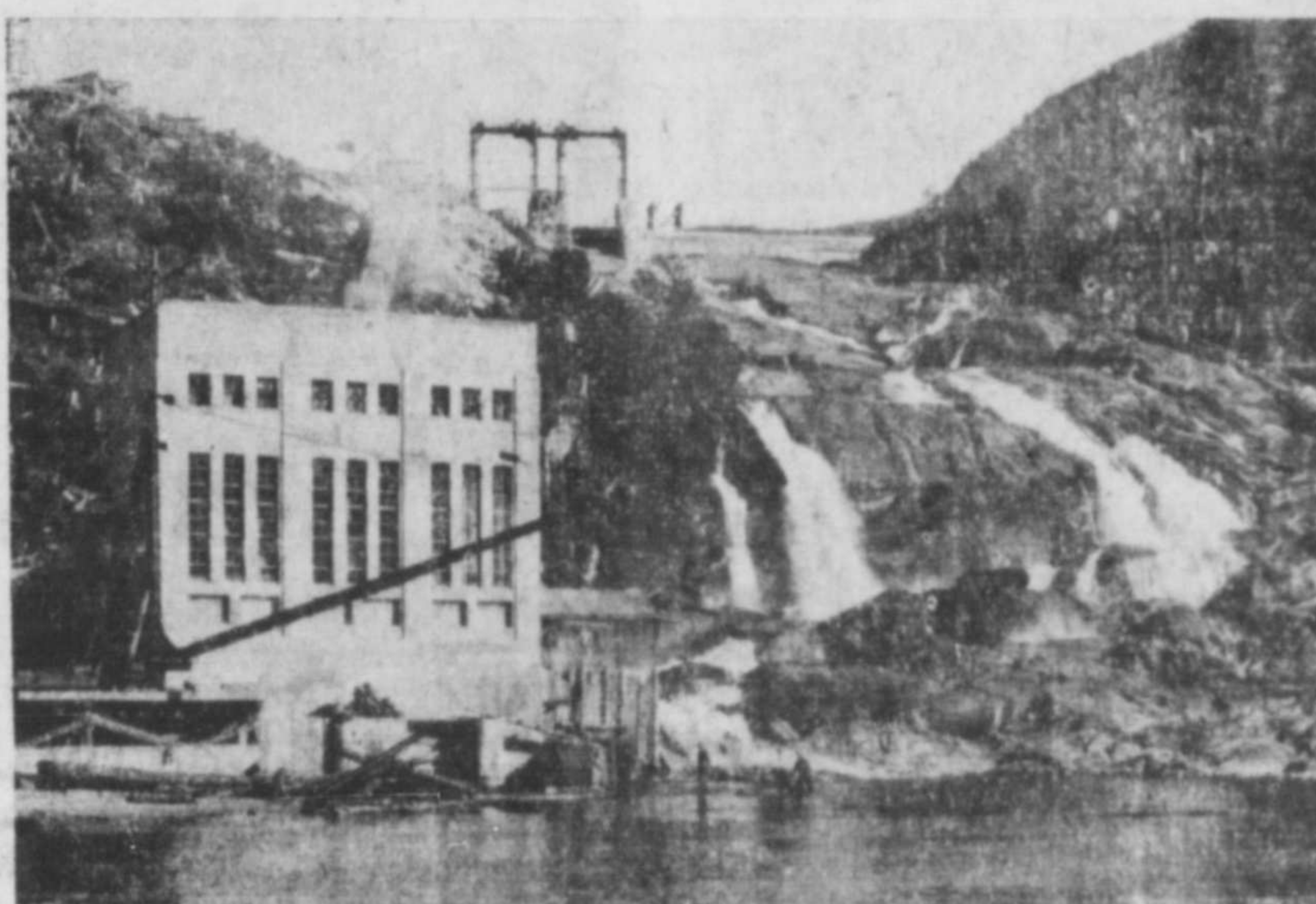
—Courtesy Electrical News and Engineering. Falls River power house in foreground with intake and sluices upstream.
