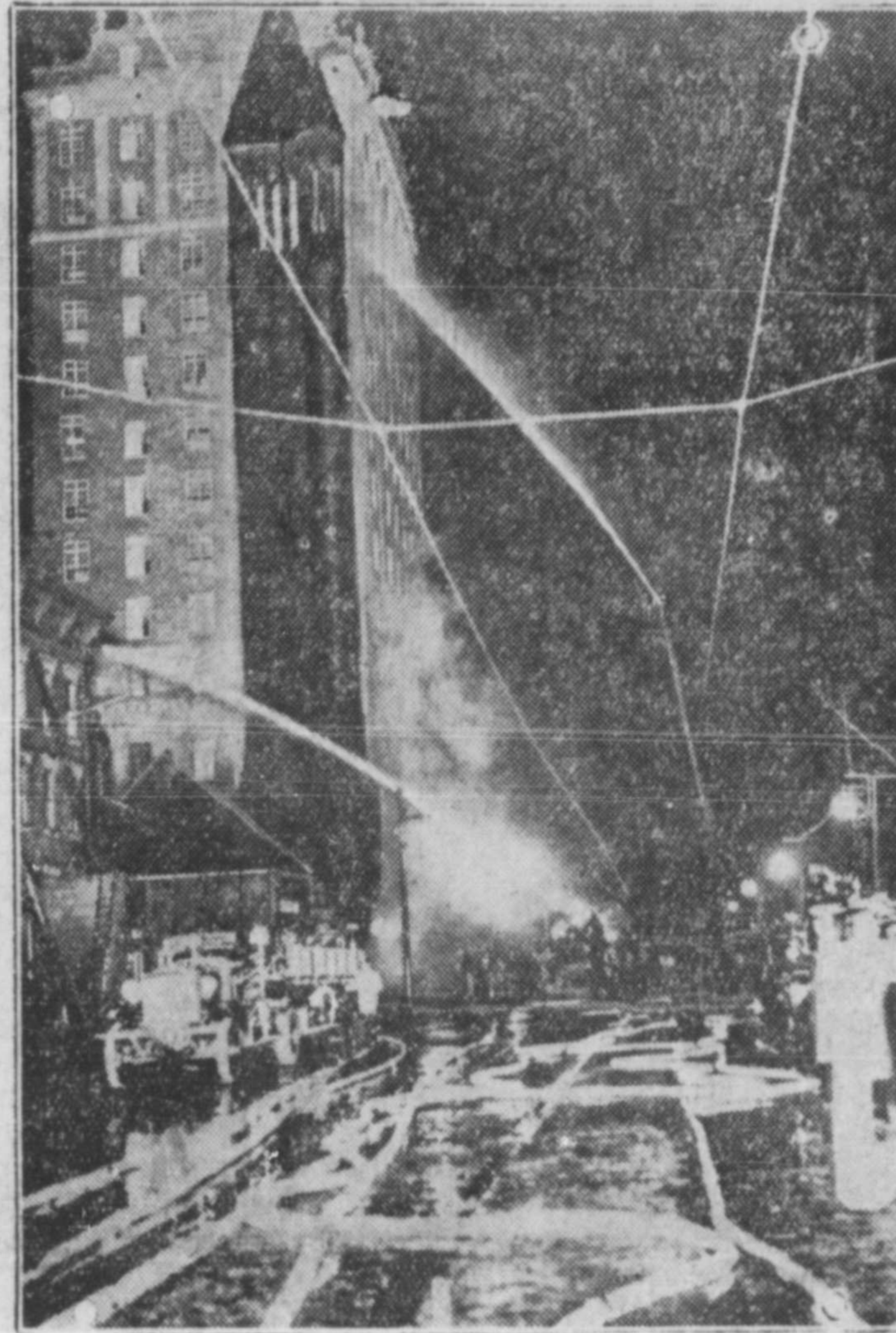
Firemen fighting devastating fire which wrecked Second Presbyterian church Newark N.J., causing damage estimated at $250,000. Four alarms called 22 fire companies into action.
