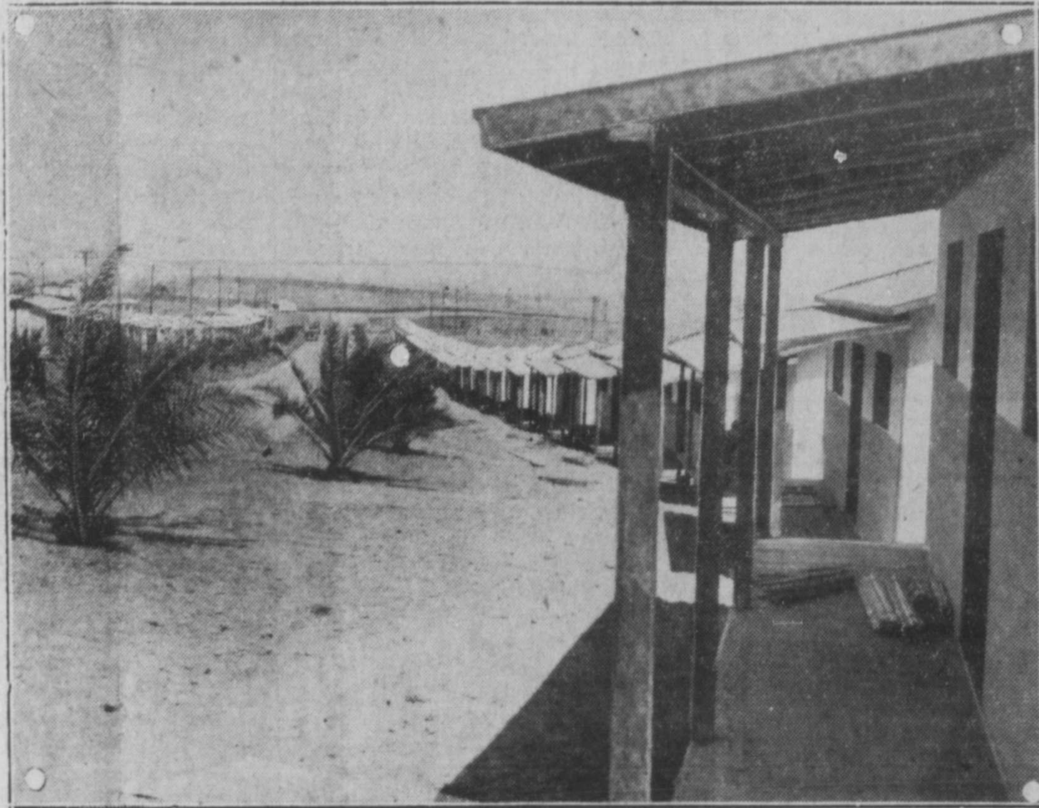
This is going to be a man's town when they finish building the tiny bungalows to be occupied by visiting male athletes who compete at the Olympiad.
