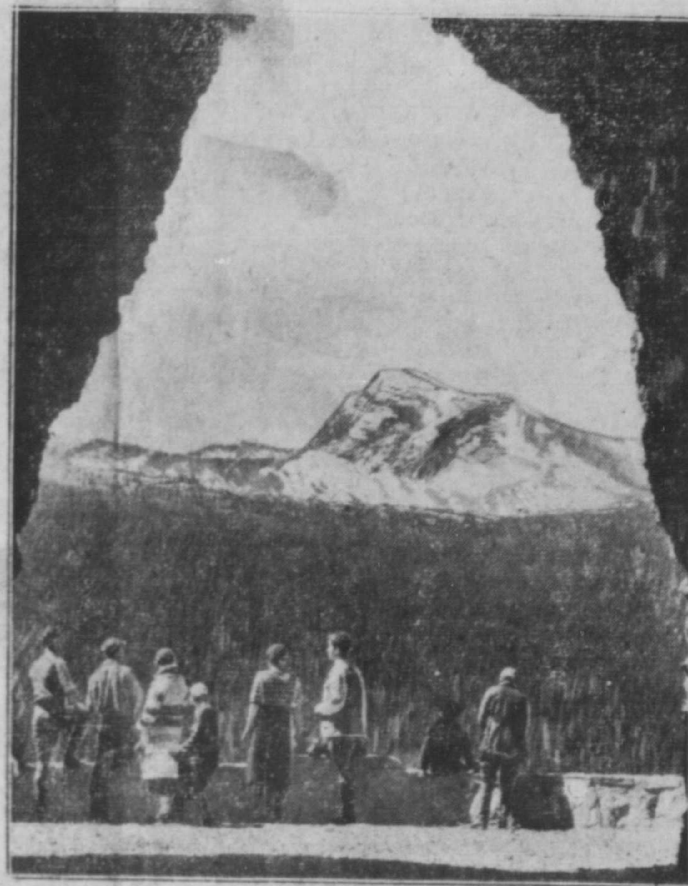
A portal in Heaven's Peak. The new Going-to-the-Sun highway soon to be opened, is one of the most scenic in America. Sky-high tunnels are lighted and ventilated by portals like this.
