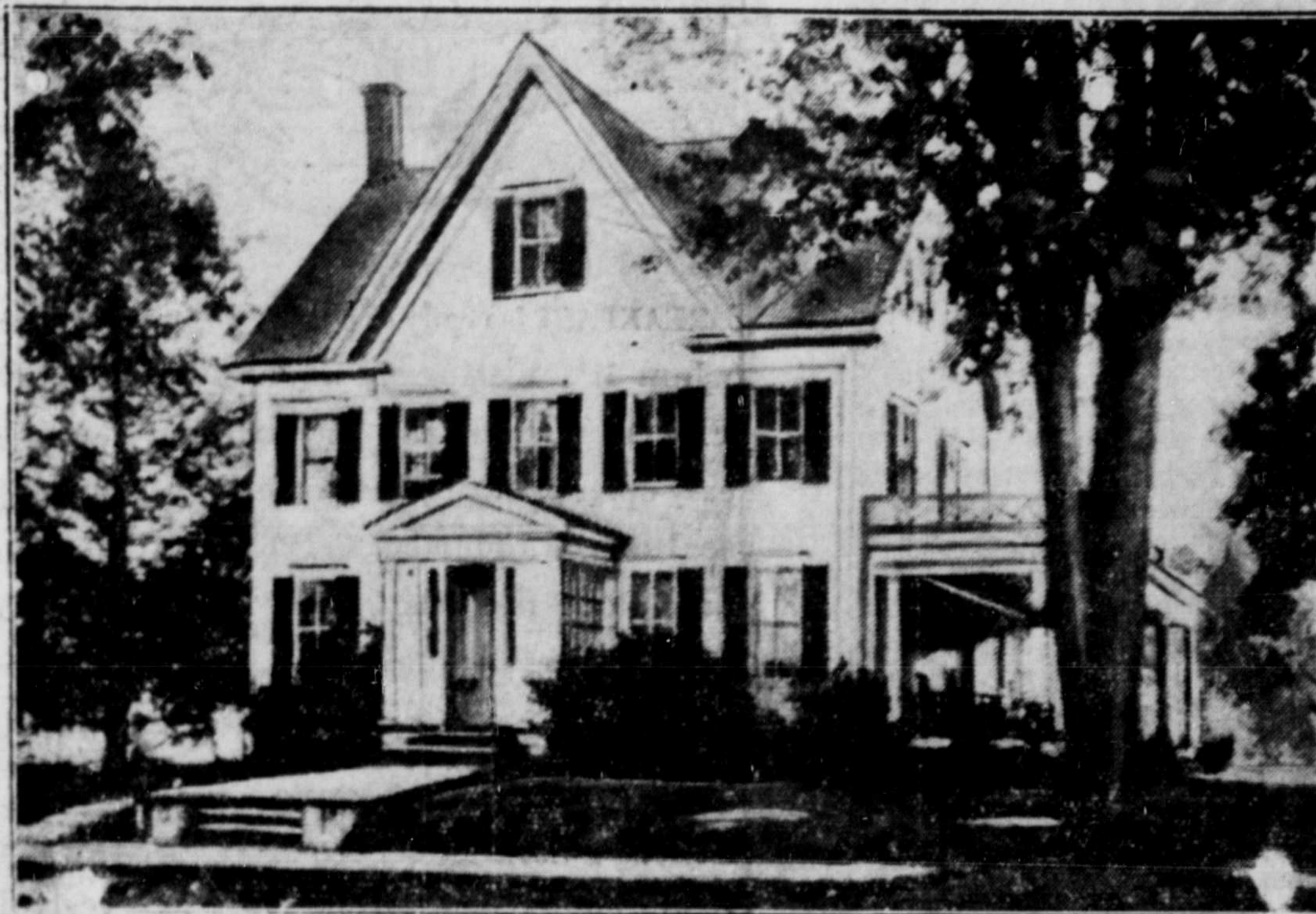
The Theta Chi fraternity house at Dartmore College, Hanover, N.H., where carbon monoxide gas killed nine students as they slept in their dormitory. A gas-connected pipe on the heating furnace in the basement permitted escape of gas. Owing to zero temperature all dormitory windows were tightly closed, which fact contributed to the fatality.
