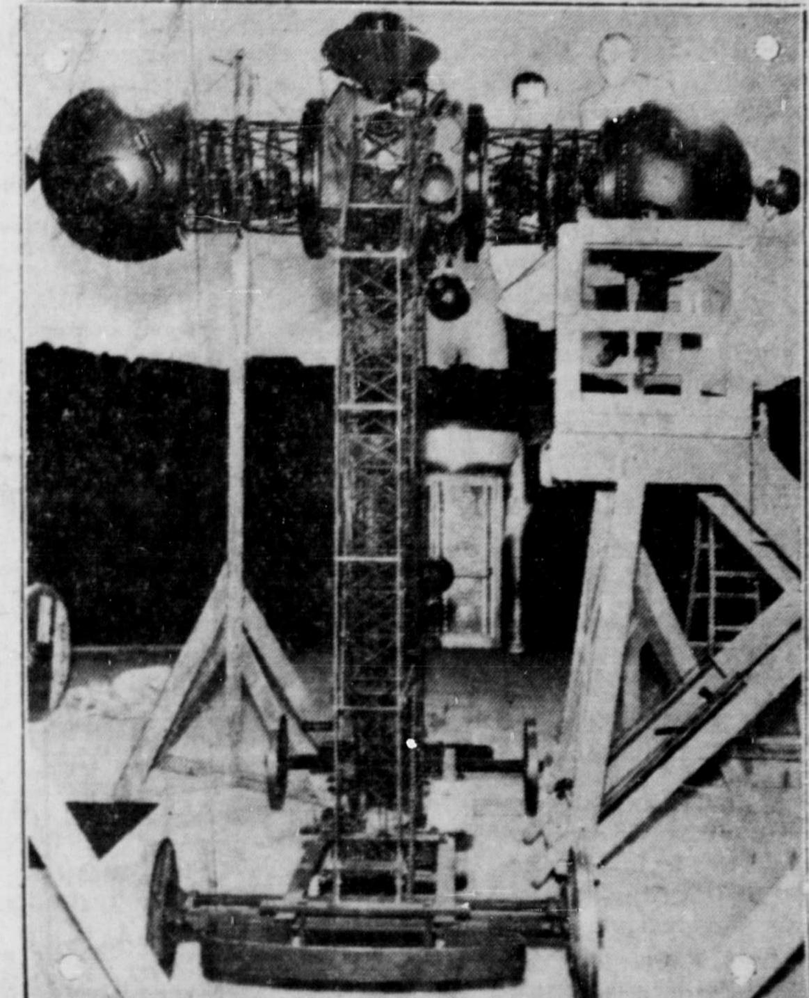
This complicated looking machi e is called a planetarium and when completed will project moving replicas of the heavenly bodies on an artifical sky in the ne Griffith observatory, at Los Angeles.
