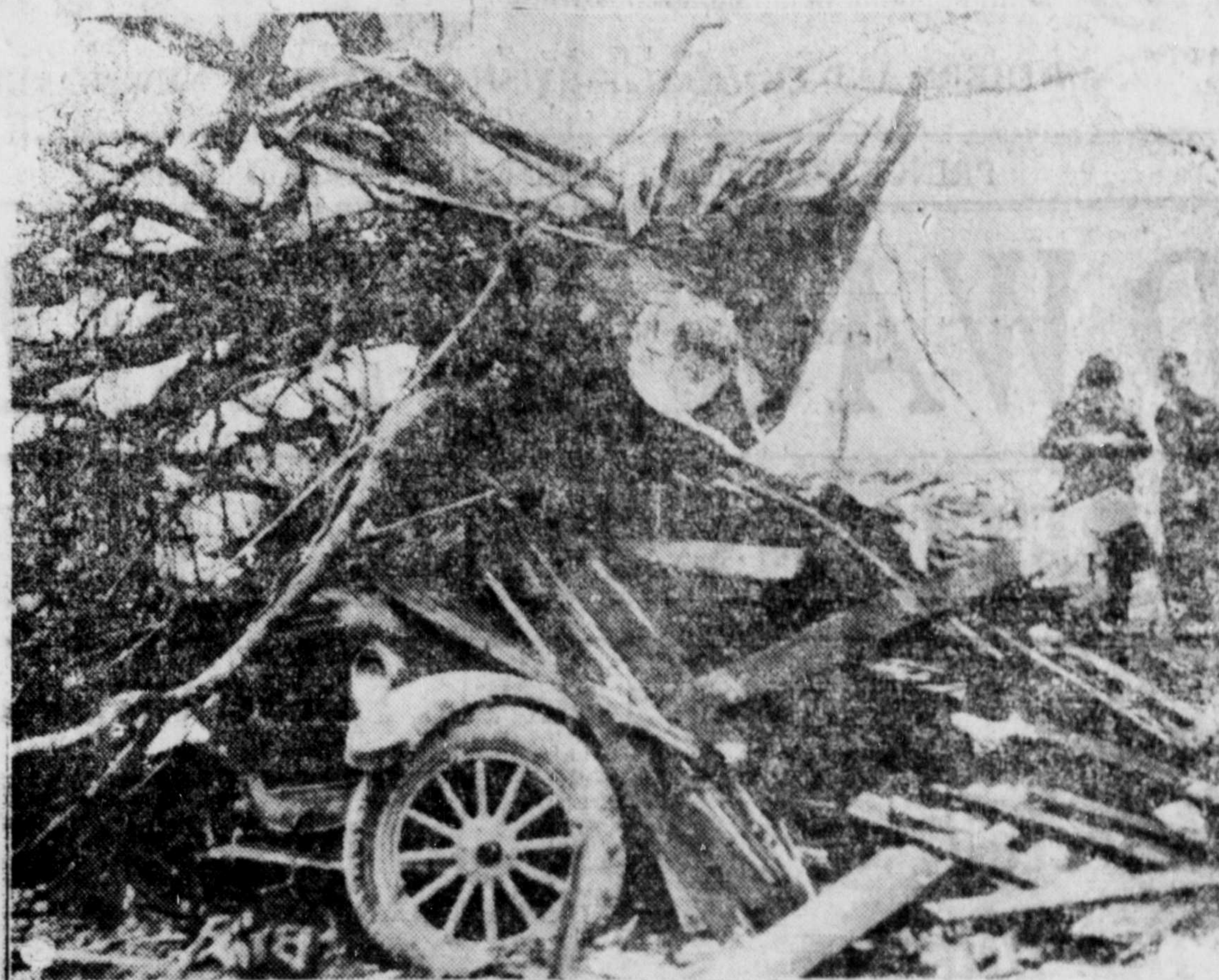
This photo shows a scene of the damage left by the madcap tornadoes which swept through Georgia, Mississippi and Alabama. The storm resulted in property damage running into the millions and caused the death of at least 23 persons, injuring hundreds of others. This picture, made in Henry county, Georgia, shows the wreckage of an automobile after a tree fell on it during storm.
