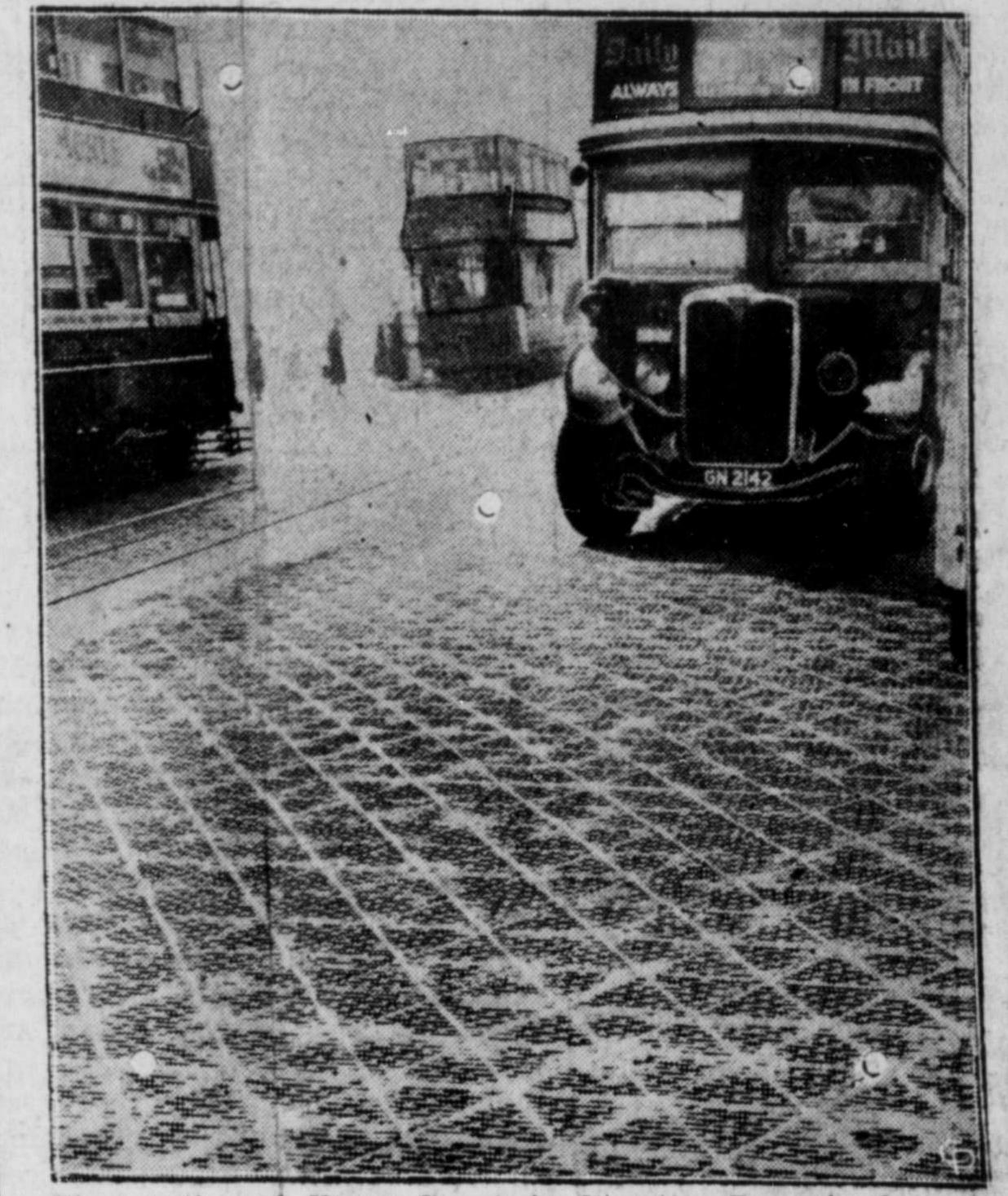
That section of Upper Street in Islington Borough, London, whereon corrugated iron street paving is being tested, is pictured. The corrugations, designed much after the style of the familiar auto tire treads, are expected to reduce skidding to the ultimate minimum, and London traffic authorities are expectant in the matter of the wearing quality of the road. They believe that in this case, surely, the familiar guarantee to "wear like iron" will
