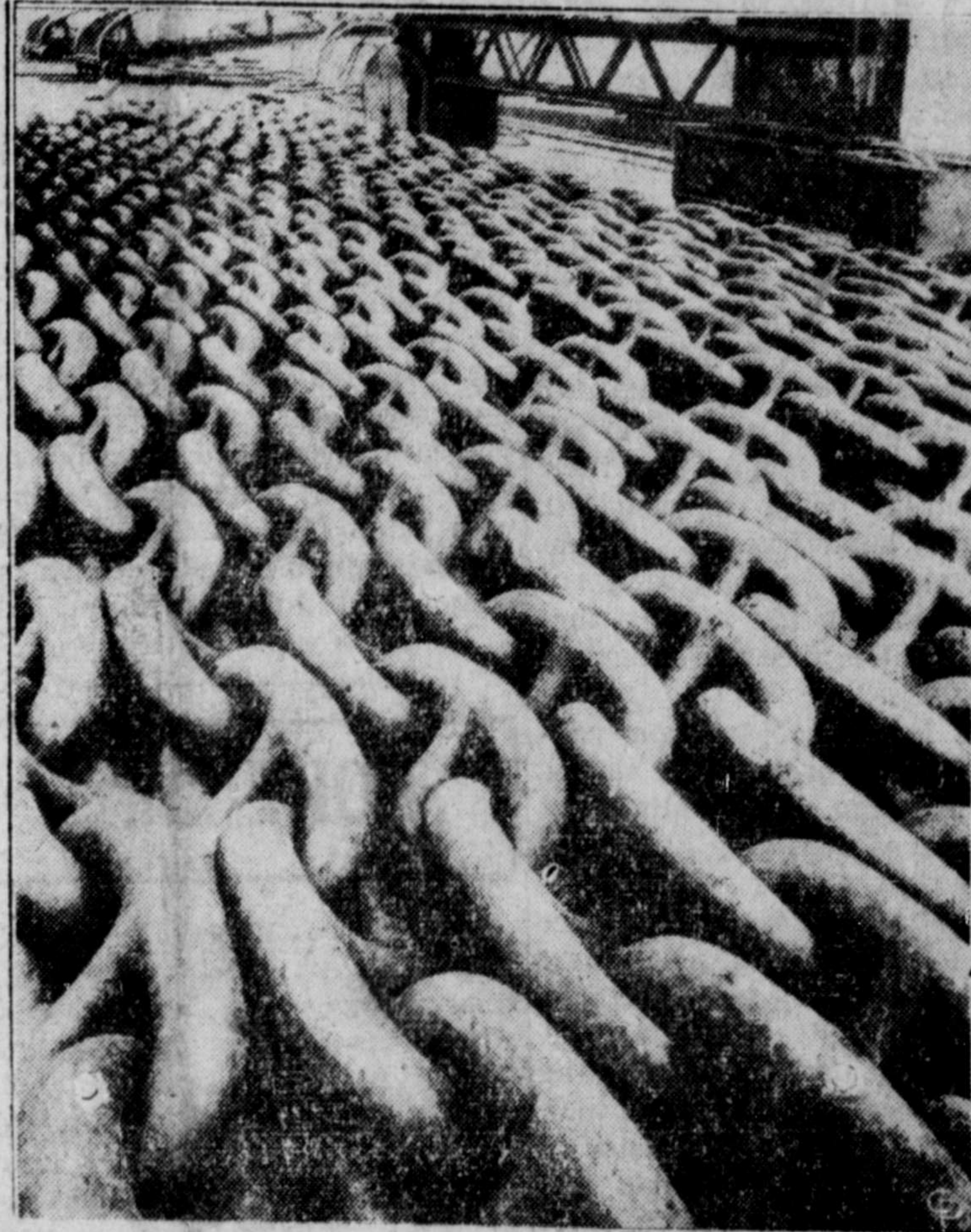
Like a tunic knitted for a giant, the links of this massive chain lie in even rows at Glasgow dock. Each link weighs 225 pounds, and is two feet in length. The 150 to 15 of anchor chain cables will be used for the Queen Mary, England's new queen of the seas.
