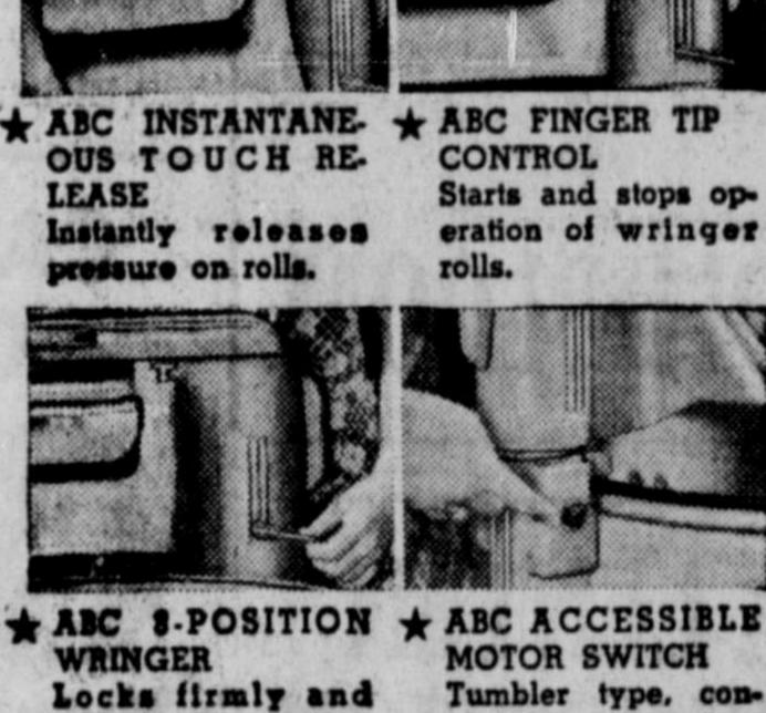
MOTOR SWITCH veniently located at the top of wringer
