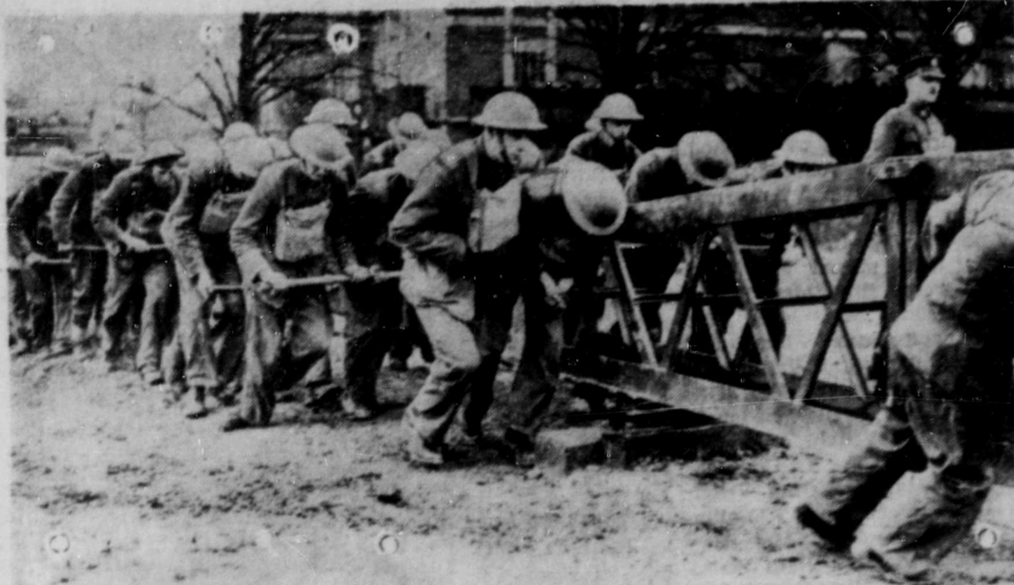
Sappers of the Royal Engineers are shown using muscle power to place a section of a steel bridge in position at an engineering school somewhere in England. Although the role of the engineering corps is primarily technical, it is a combatant arm and trained in the use of rifle and bayonet as well as transit and micrometer.
